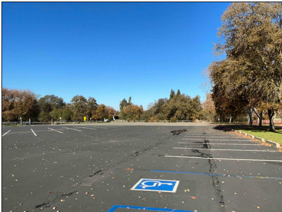
Photo D-10. View looking northwest from southeast corner of parking lot, east of Bridge Road.
