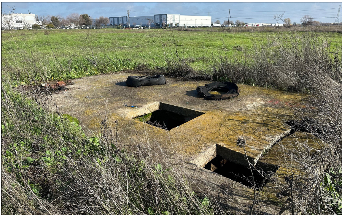
Photo 8. View of abandoned structure within Study Area; facing northeast. Photo taken 1/17/24.
