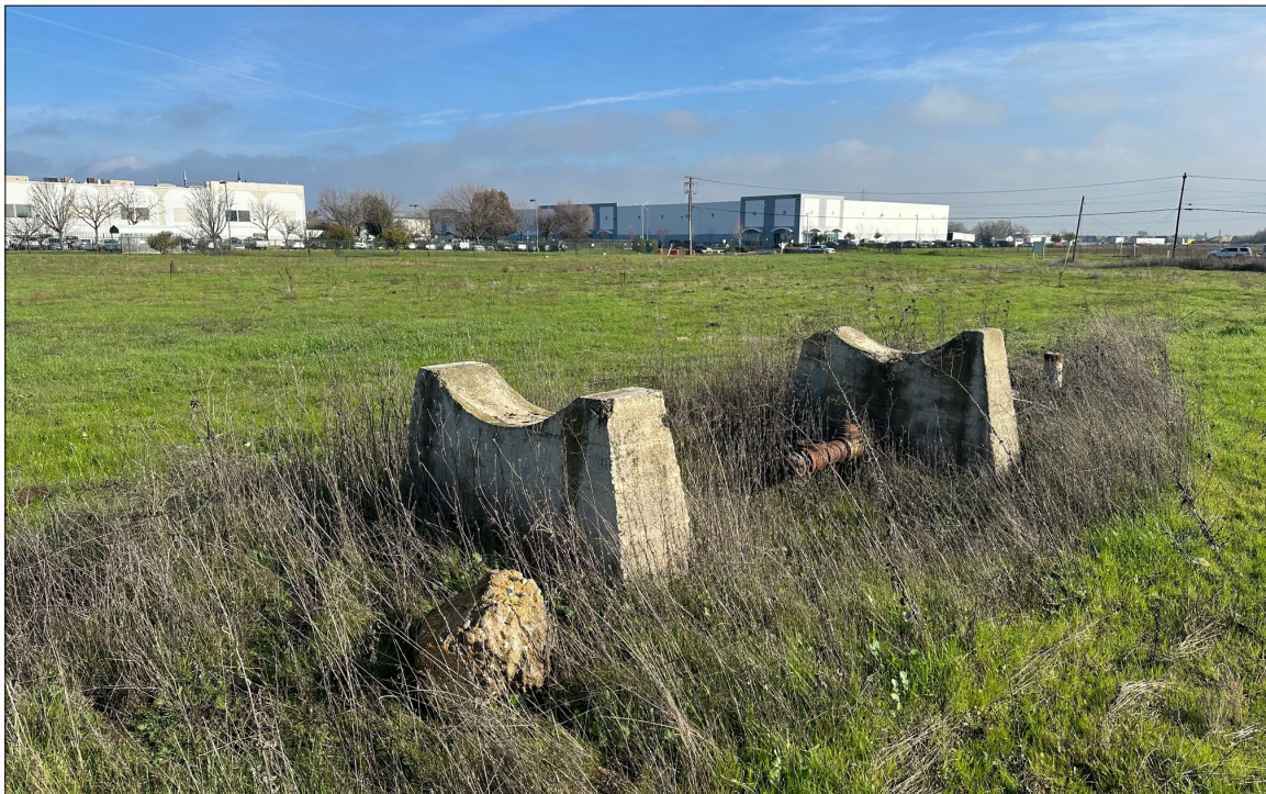
Photo 7. View of abandoned structure within Study Area; facing northeast. Photo taken 1/17/24.
