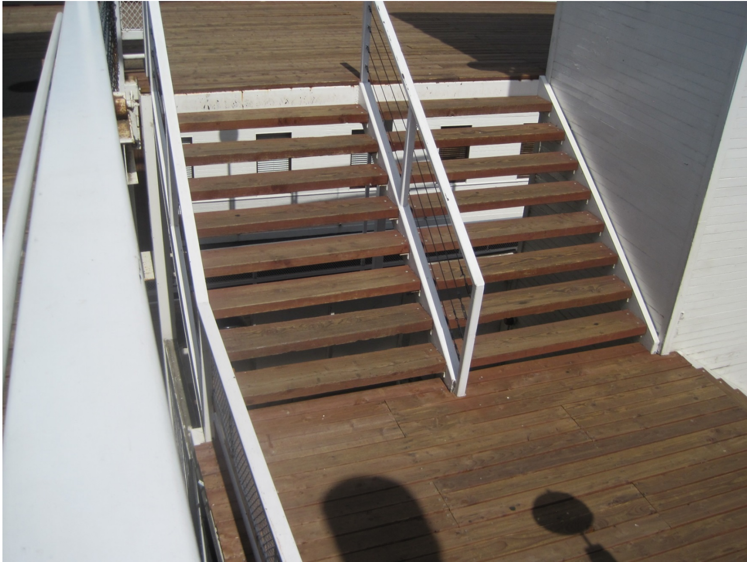
Figure 10: Current Condition of the Stairs.
