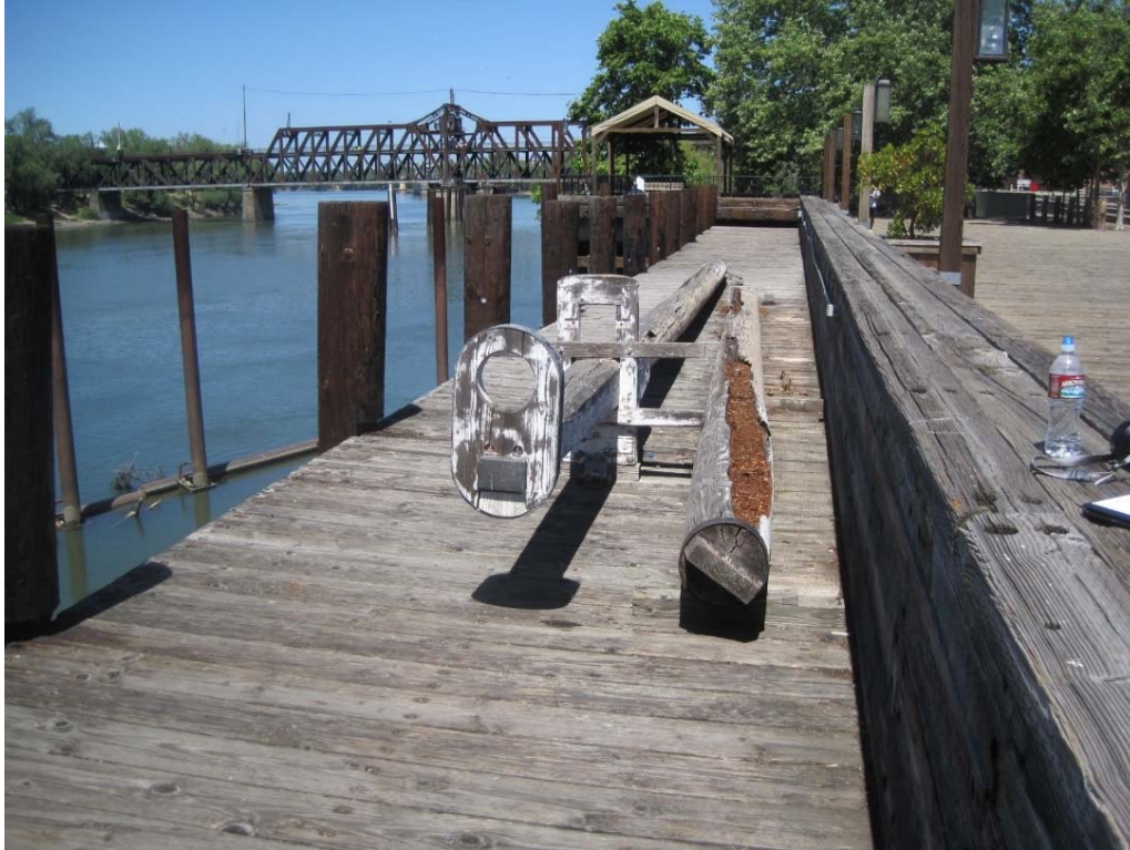
Photograph 1-6: Cantilevered Pier Section at North End of Project
