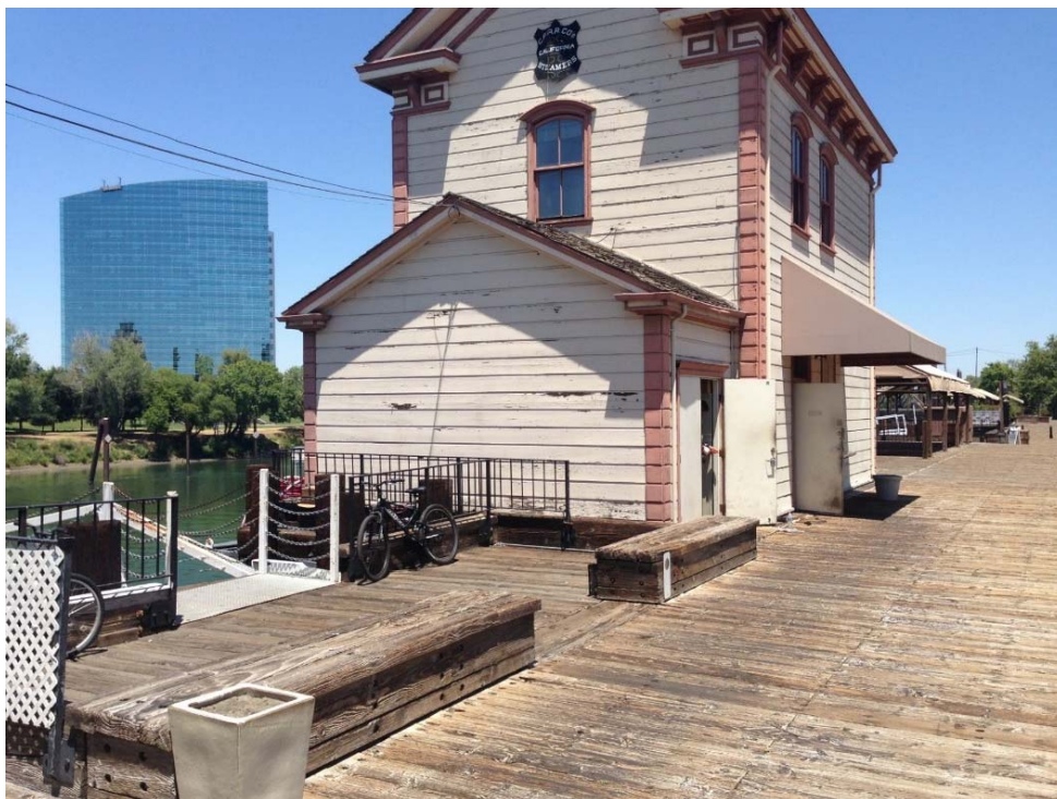
Photograph 1-8: One-Story Addition on California Pacific Steamers Building
