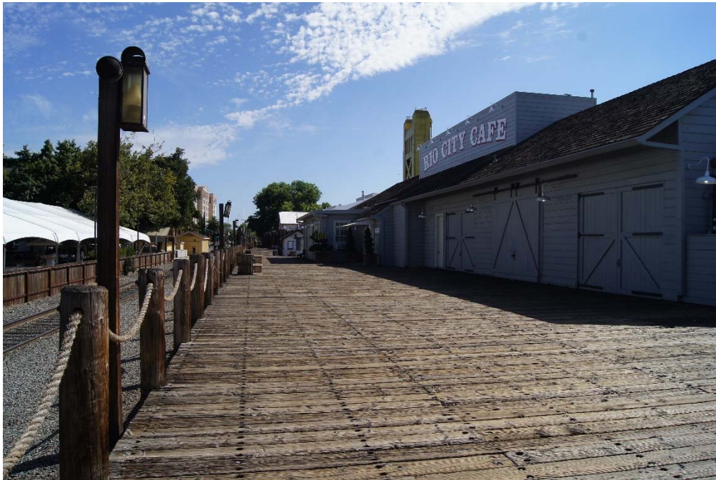
Photograph 1-1: Overview of Existing Old Sacramento Embarcadero Bolted Wood Surface, Looking South
