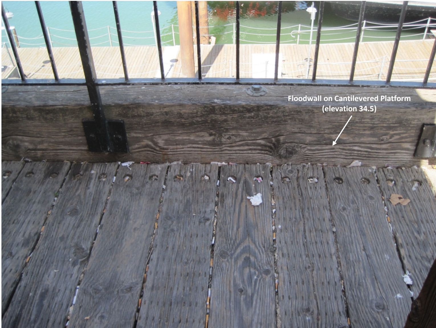
Figure 8. Timber Beam that Forms the Floodwall on the Elevated Embarcadero Sections.
