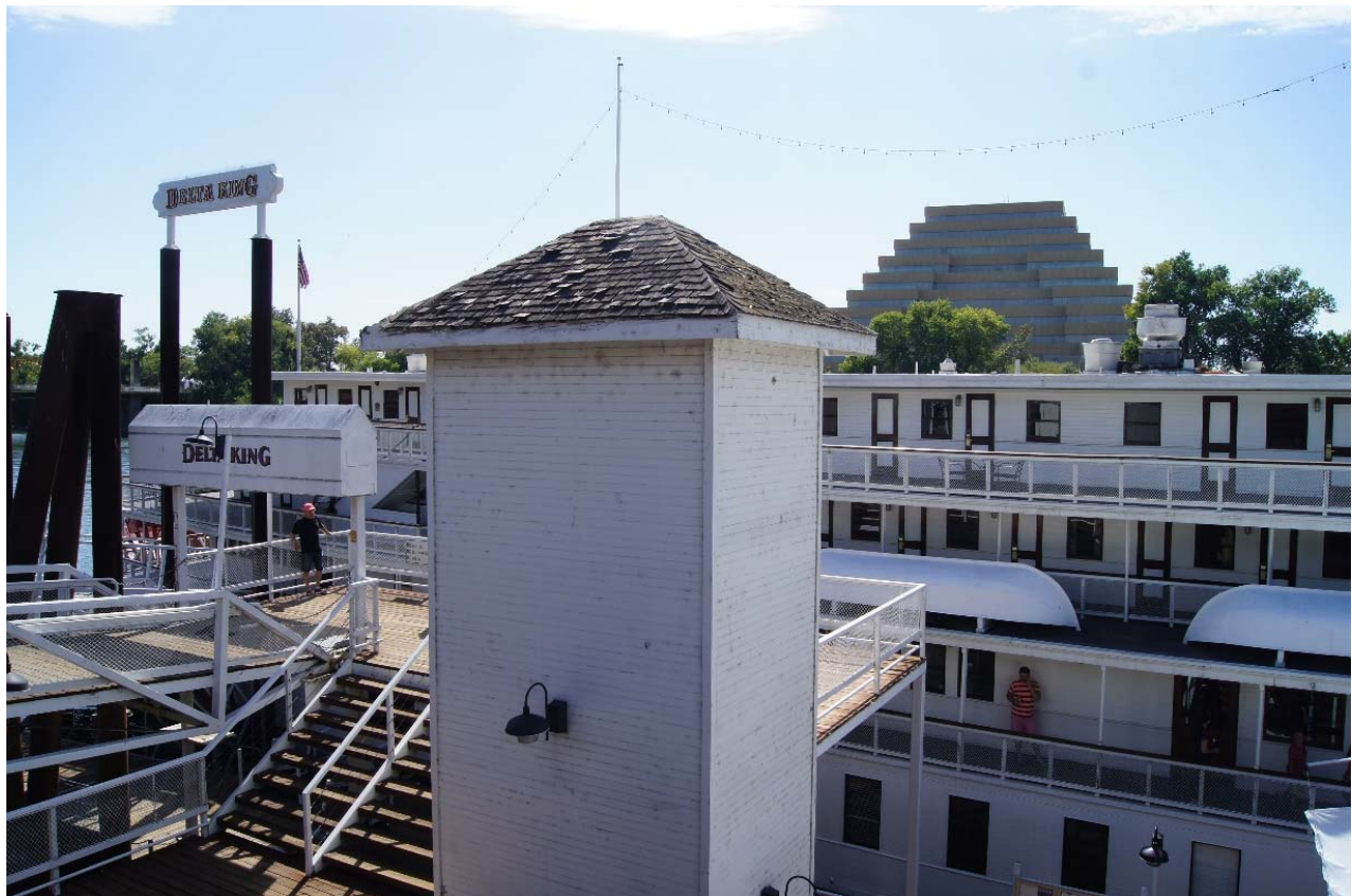
Photograph 1-5: Hoistway and Elevator Accessing Delta King, Facing Southwest
