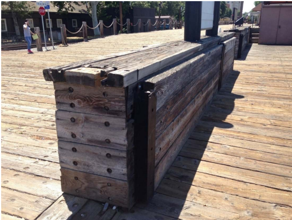
Photograph 1-2: Representative Floodwall Section
