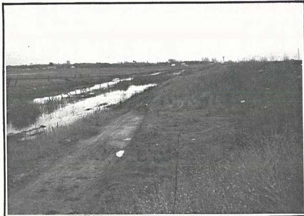
Canal and berm, view to south at Sorrento Road intersection
