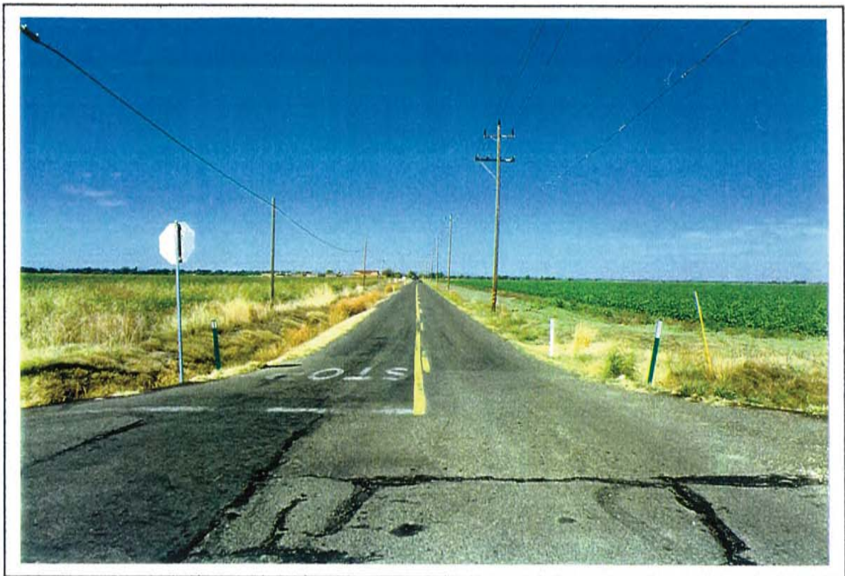
Del Paso Road; view to west from El Centro Road.
