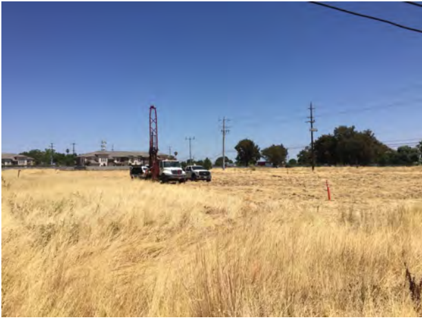
1. View of the Subject Property looking Northeast.
