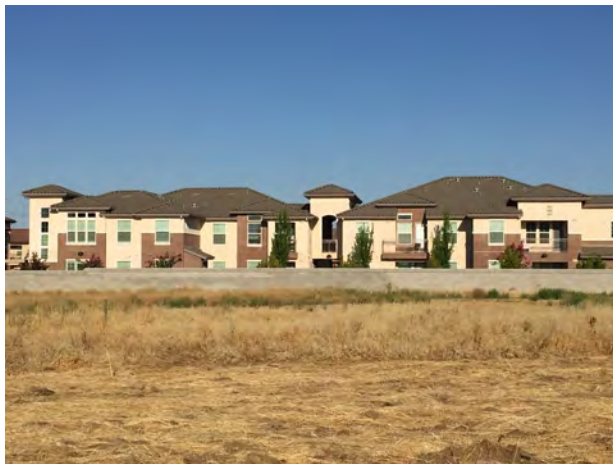
3. View of the north-central portion of the Subject Property looking North.
