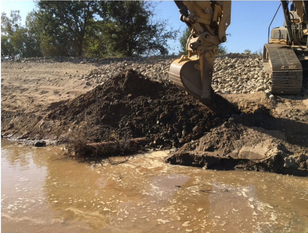
Figure 2-3. Example Woody Material Placement -Sacramento Bar, 2016
