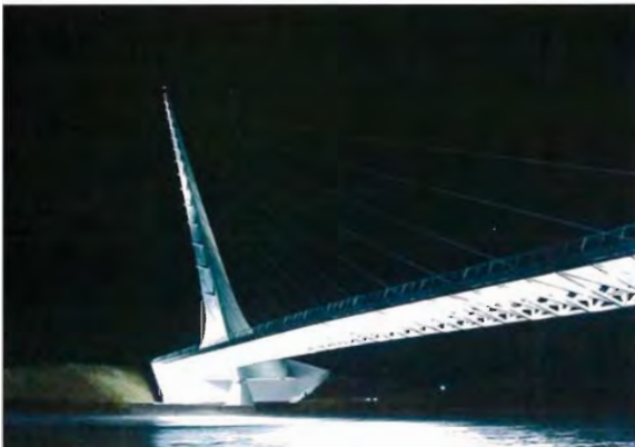
Photo 6. Nighttime lighting of the Sundial Bridge with significant illumination of the Sacramento River.
