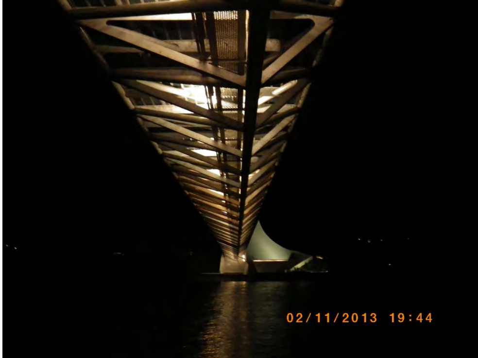
After shot of the Sundial bridge showing reduced lighting
