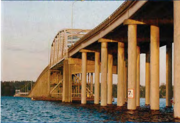
SR 520 Bridge – west end
