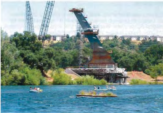
Photo 1. Sundial Bridge under construction.
