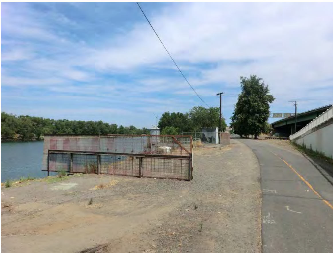
Photograph 9. Sacramento River East Levee at a location south of the proposed new bridge.
