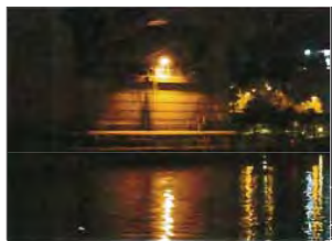
FIGURE 50. Artificial lighting under the University Bridge. Lighting is directed down onto the water surface. Light on the north bridge support structure is pictured. Light on the south support structure is similar. These lights correspond with green circles in Figure 47.
