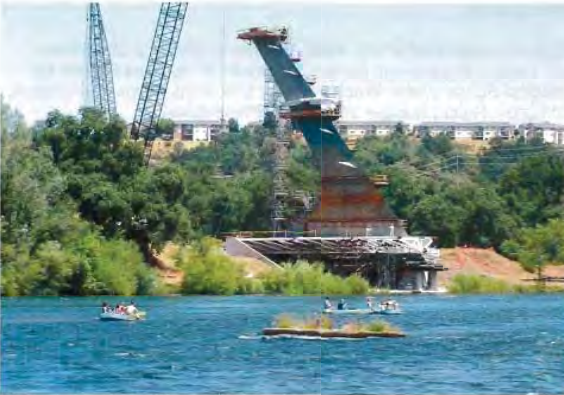
Photo 1. Sundial Bridge under construction.
