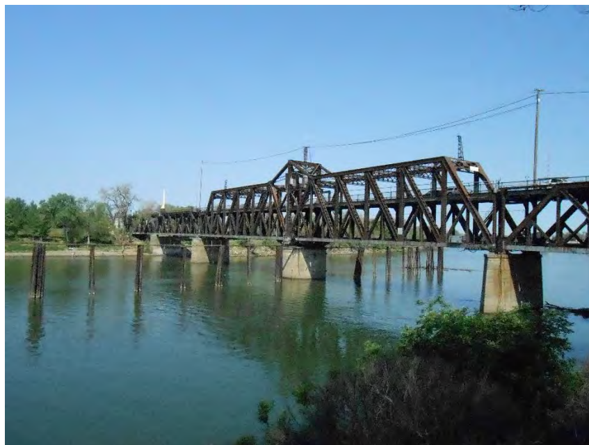
Photograph 1. General view of I Street Bridge from Old Sacramento.
