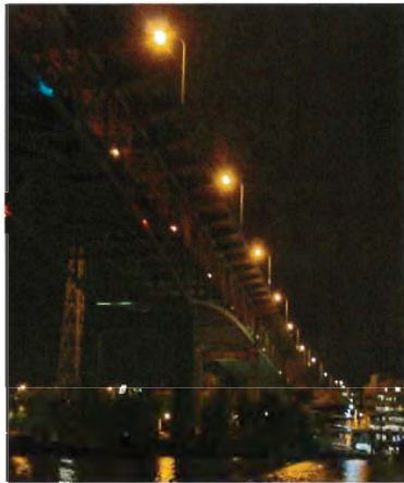
FIGURE 48. Artificial lighting on the I-5 bridge deck spanning the Lake Washington Ship Canal (looking north).
