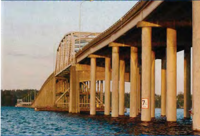
SR 520 Bridge – west end
