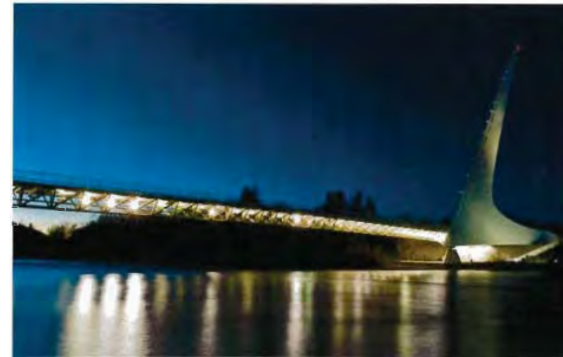
Photo 4 – Sundial Bridge lit up at dusk, with lights pointing down towards the Sacramento River, in a downstream direction.
