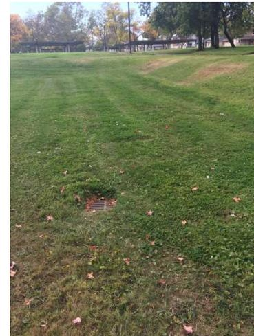
Photo 4. Drain located within depression feature
