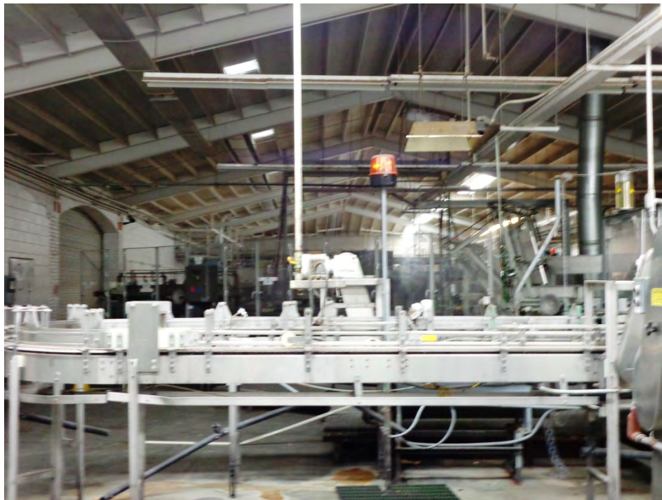
Production Building (west courtyard wing)
