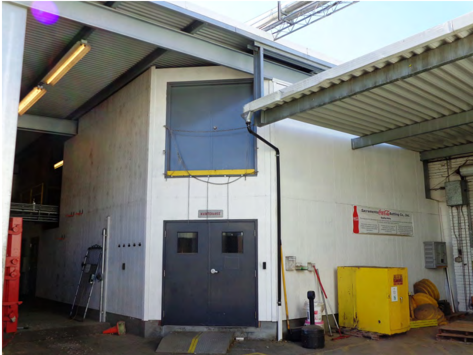
Maintenance Building (non-contributing)
