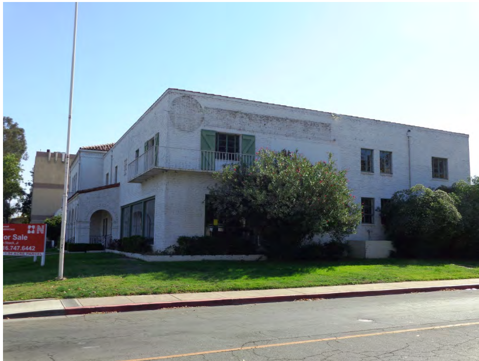
Northern Elevation of Administration Building
