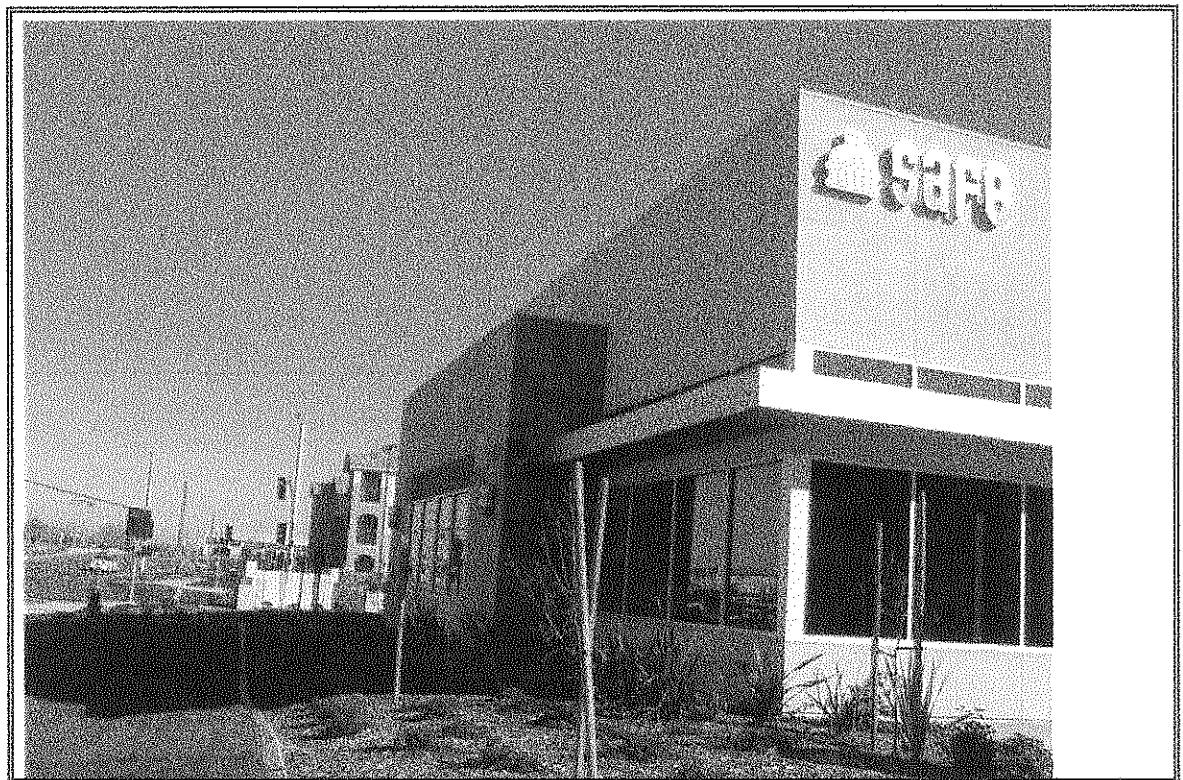
Photograph Number 6 West side of 2200 Building
