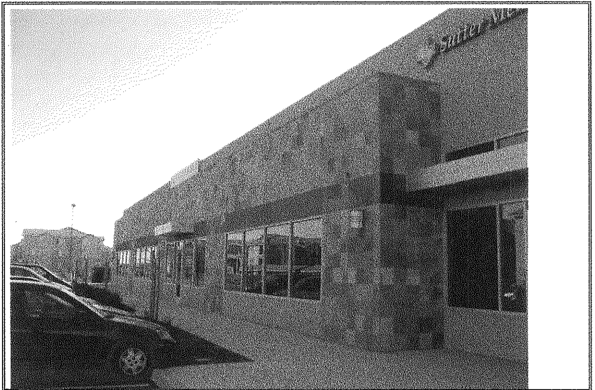
Photograph Number 15: East side of 2210 Building
