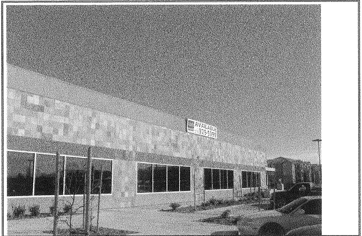
Photograph Number 5: West side of 2210 Building
