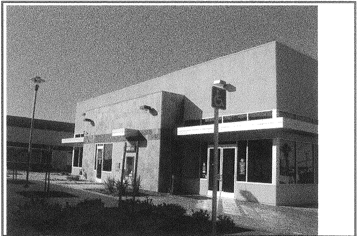
Photograph Number 16 South side of 2200 Building
