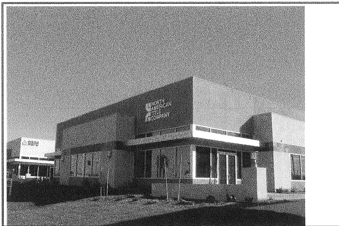
Photograph Number 8 Northwest side of 2230 Building
