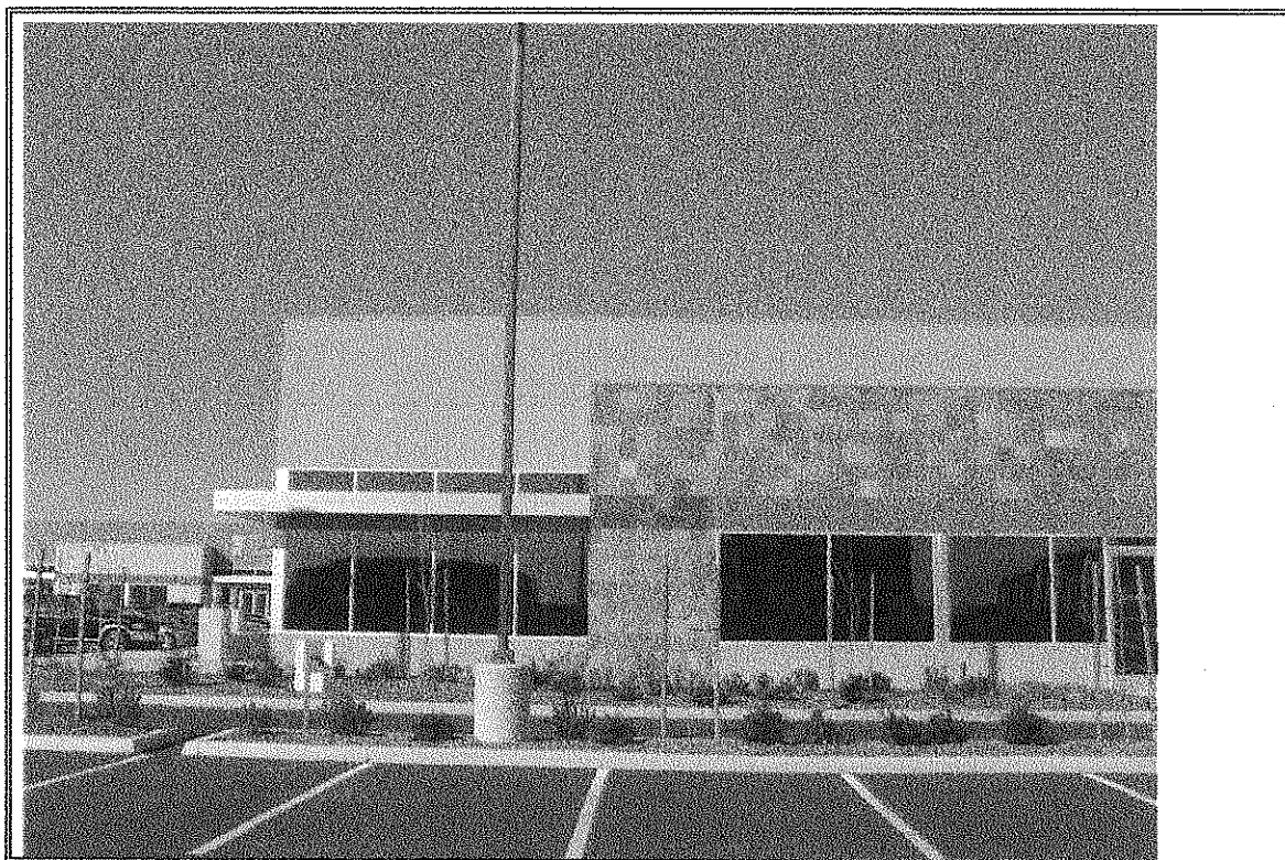
Photograph Number 2 South side of 2210 building
