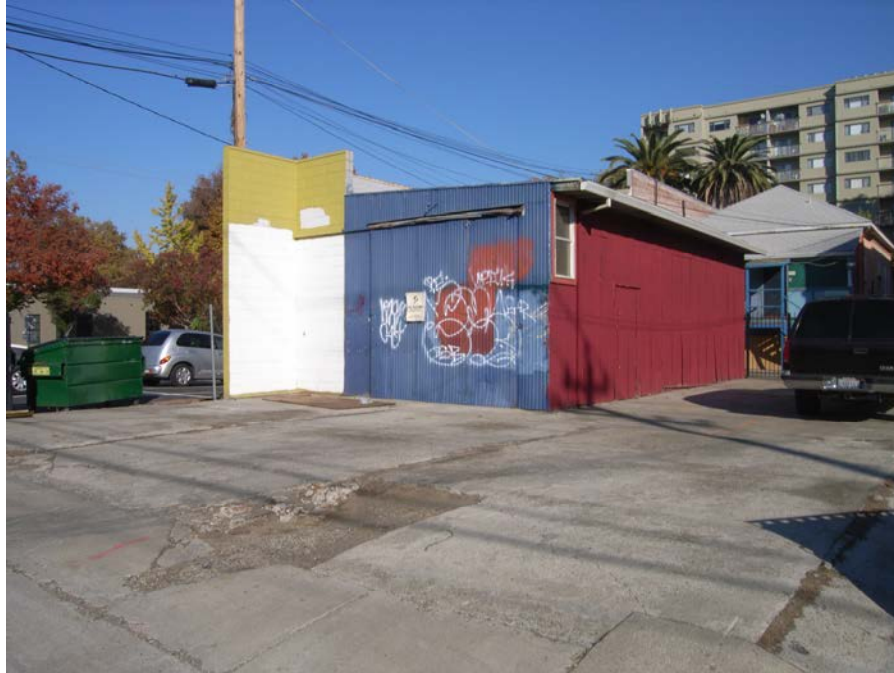
Photograph 5. Building 2, camera facing northwest
