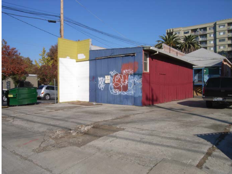
Photograph 5. Building 2, camera facing northwest
