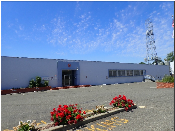
Photograph 23. 76 Broadway - Phillips 66 office building (#20) (view to south)
