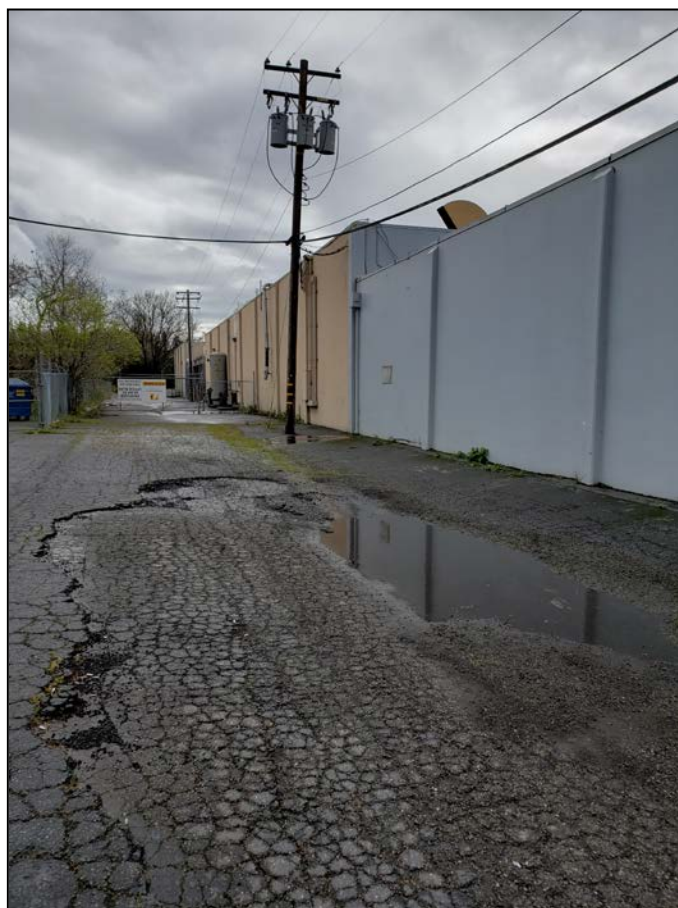
North side of building, view to east
