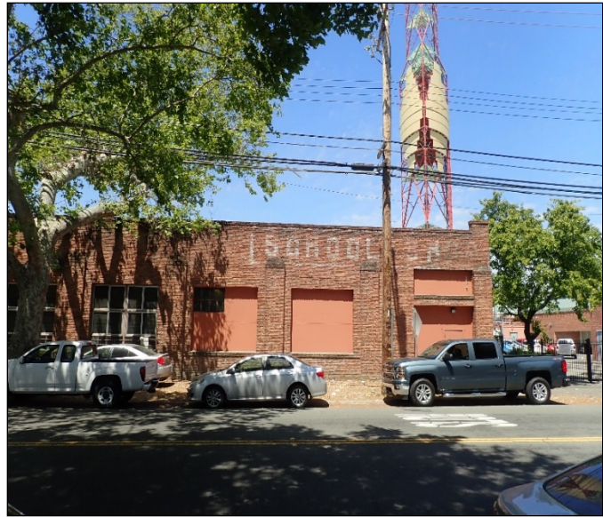
Photograph 12. 425 1 st Ave. - SCUSD Operations Center (#9) (view to south)
