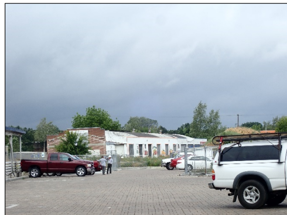
Photograph 7. P-47-03382 Farmers Market building segment adjacent to 3 rd St. (#3b) (view to west)
