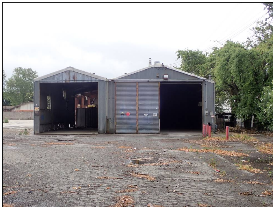
Front view of storage sheds, view to east
