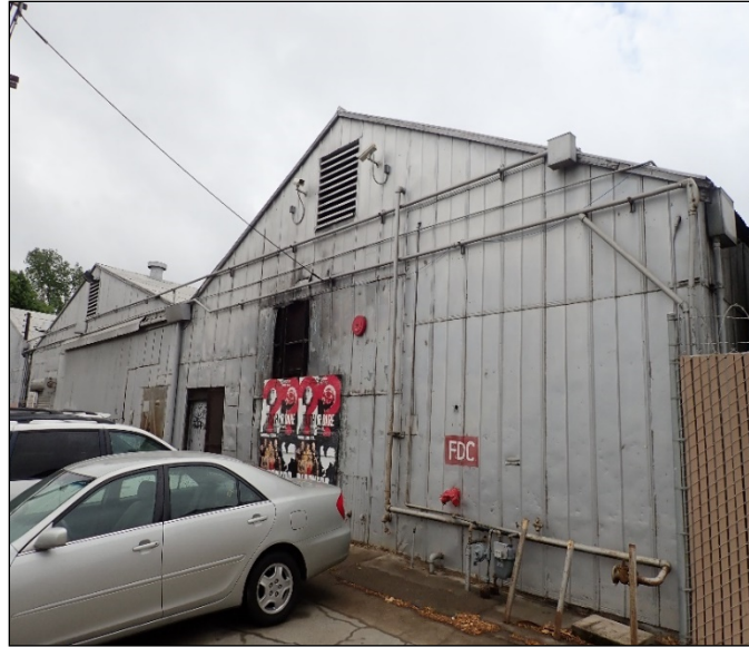
Photograph 20. 600 1st Ave. (abandoned warehouses) (#17) (view to southeast)
