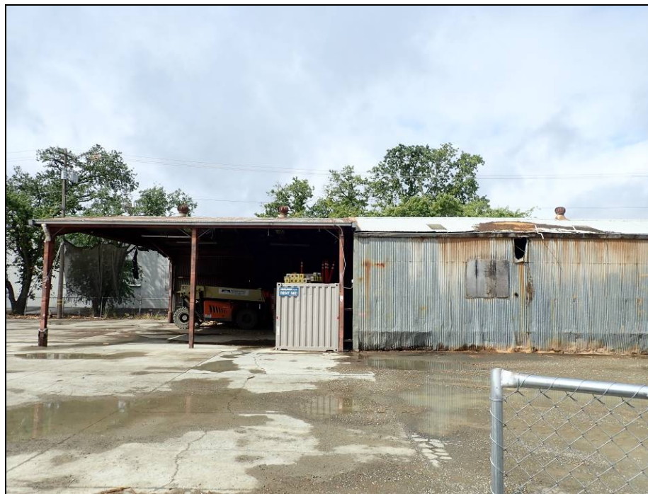
Side view of metal storage sheds, view to south
