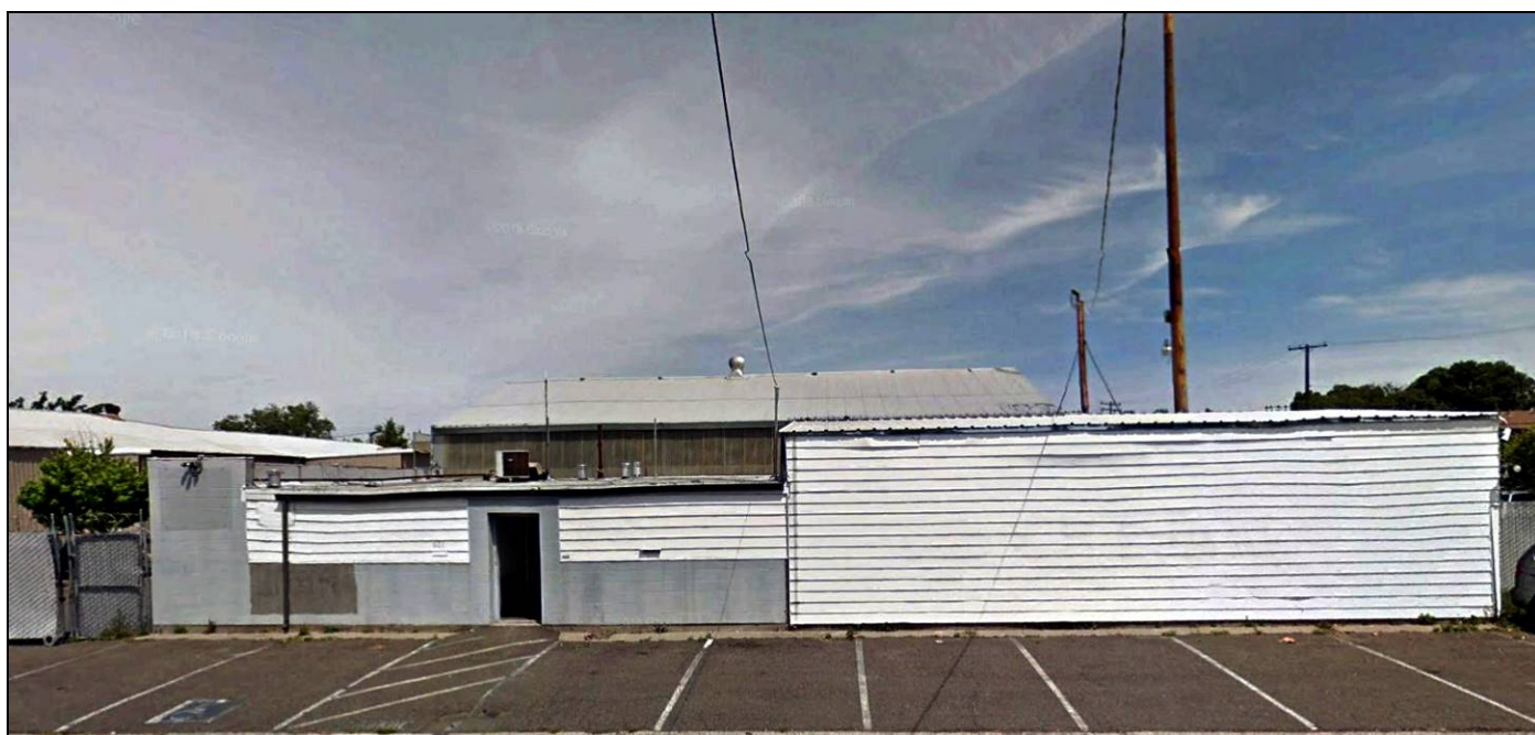
Overview of three corrugated metal buildings, view to north
