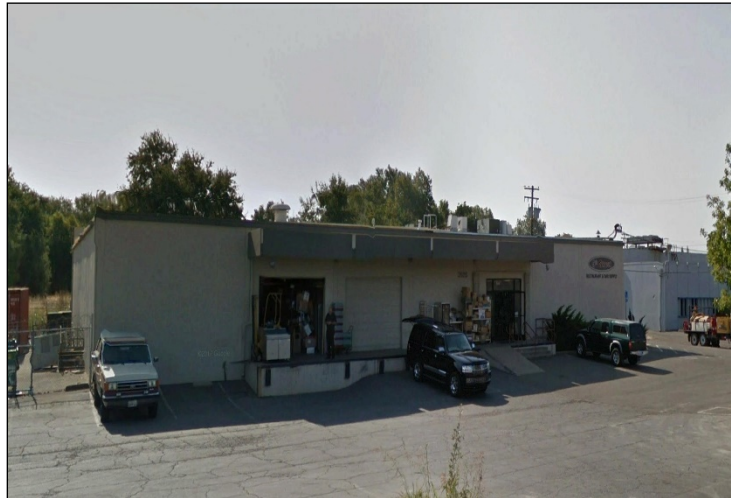
Photograph 17. 2625 5 th St. - 5 th Street Restaurant & Bar Supply (#14) (view to east)
