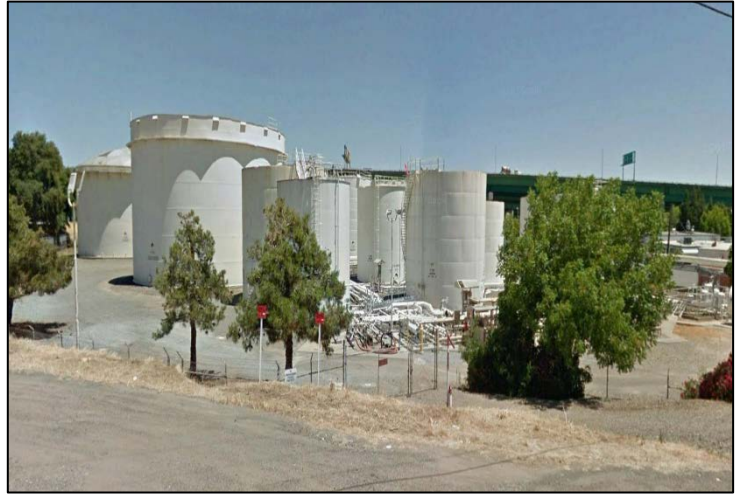
Photograph 24. 2420 Front St. - Chevron Bulk Terminal (#21) (view to north)
