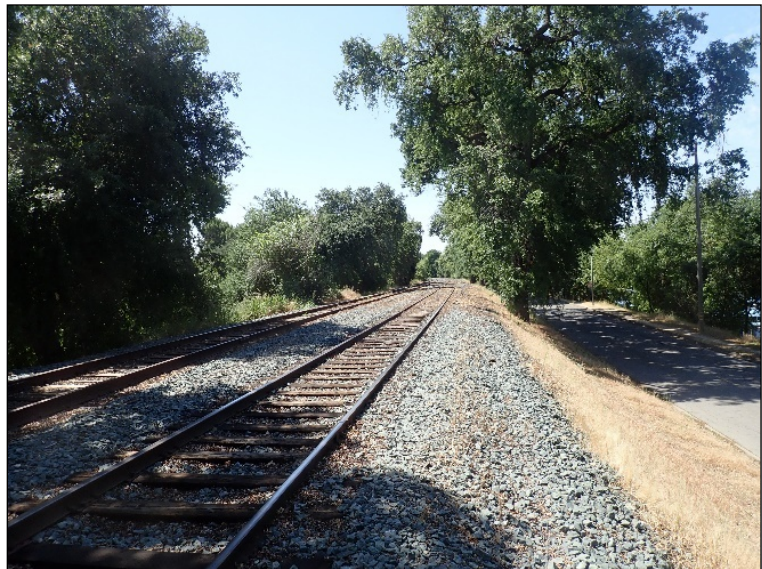
Photograph 5. P-47-01497 double track (#2) (view to south)
