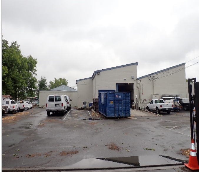
Photograph 14. 2535 5 th St. - SCUSD Business Center (#11) (view to north)
