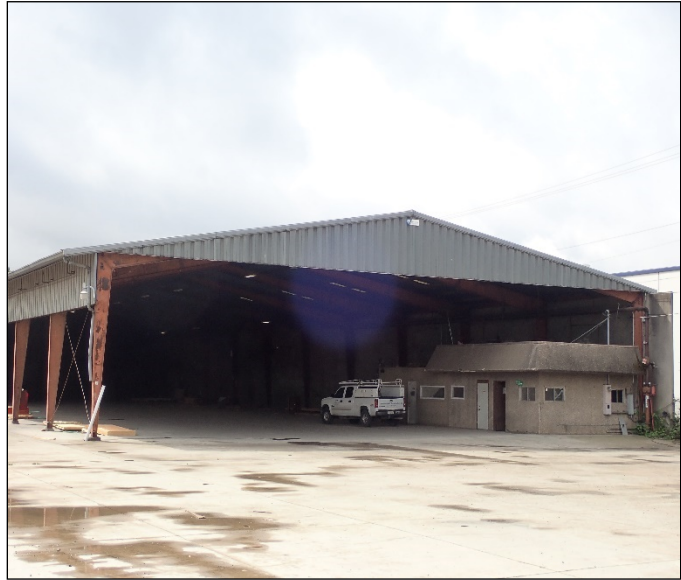
Photograph 18. 2681 5 th St. - Pacific Pallet Exchange (#15) (view to southwest)
