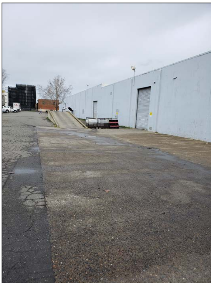
South side of building, view to west
