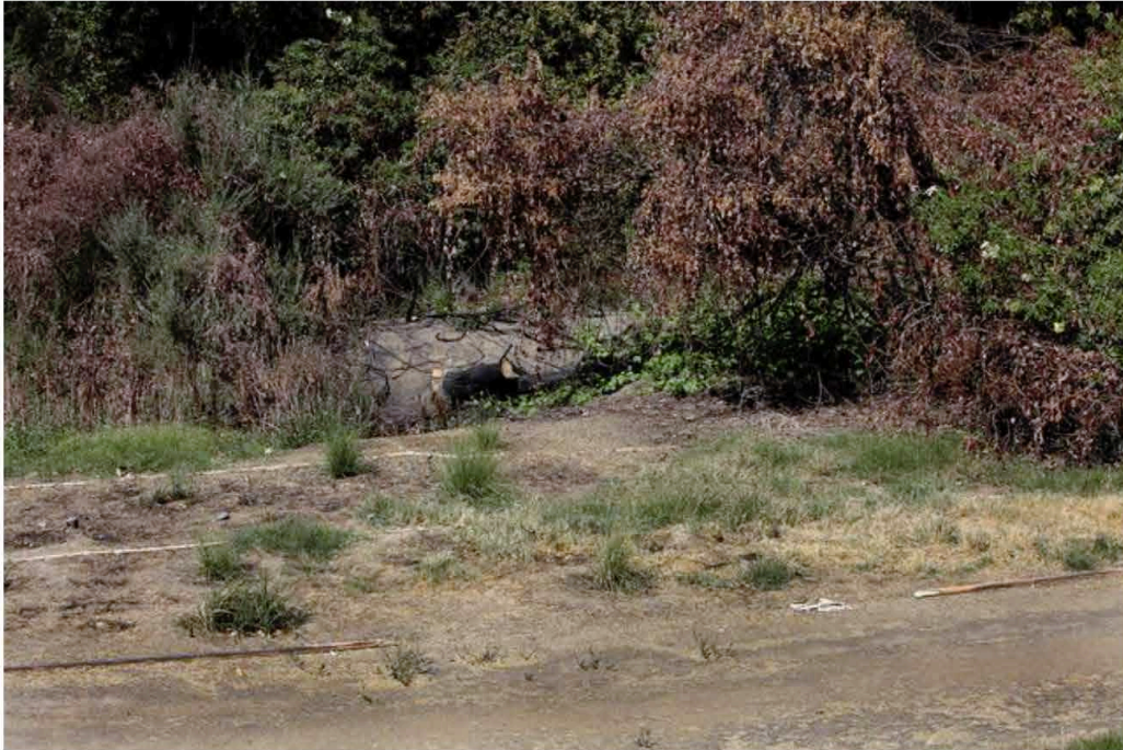
Photo 1. Evidence of a fire directly adjacent to the existing Sutter's Landing portion of the Two Rivers Trail. Environmental plantings are in the foreground with broken irrigation lines.
