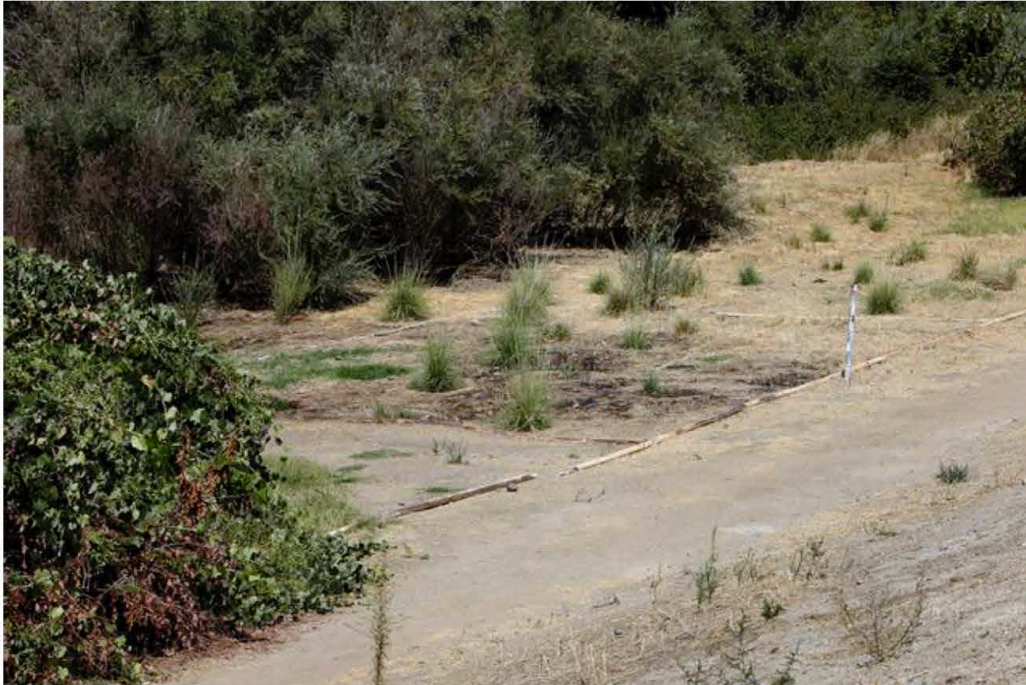
Photo 2. Environmental restoration plantings with broken irrigation lines along the existing Sutter's Landing portion of the Two Rivers Trail. Were these accepted by the regulating agencies as adequate mitigation measures and are these still being monitored?
