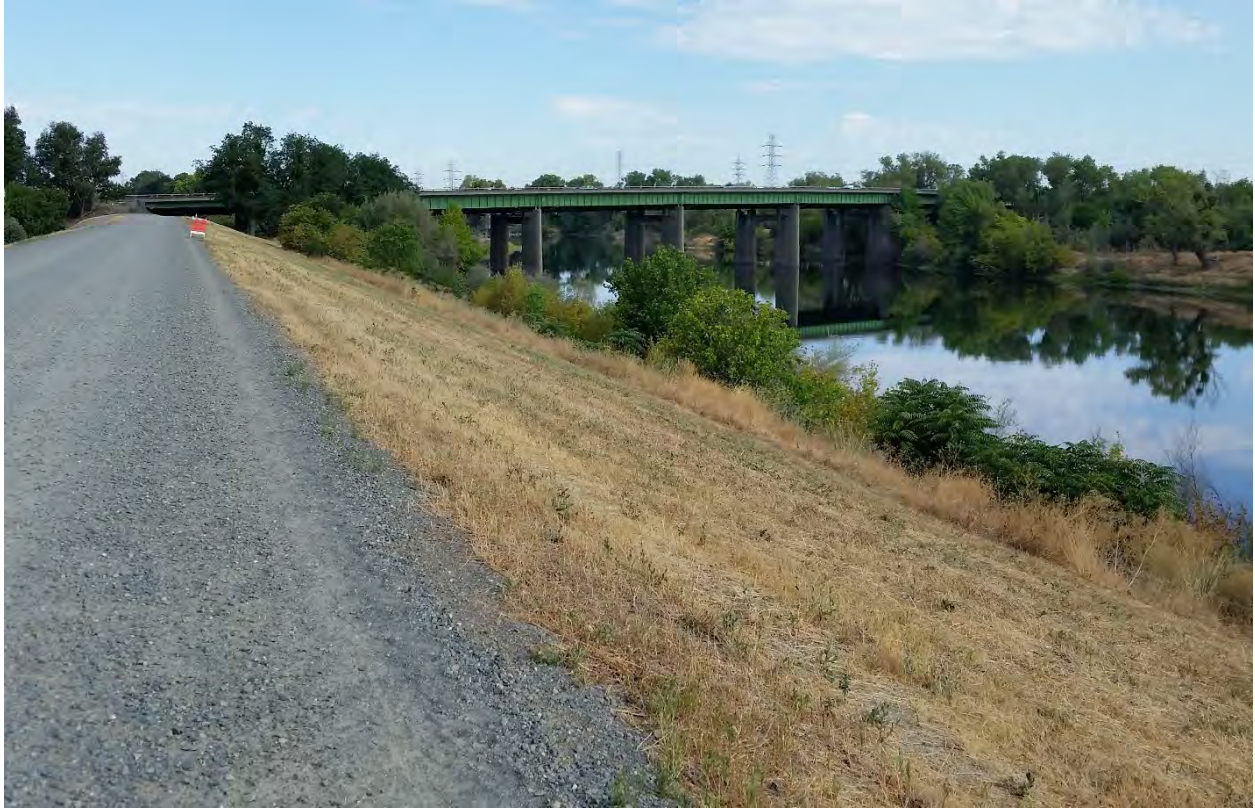
Photo 3: Facing west towards Business 80 bridge. The proposed trail would be on the slope of the levee here due to the lack of levee toe road.
