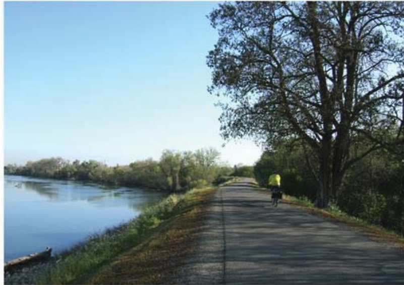
Recreational multi-use path along the Sacramento River.
