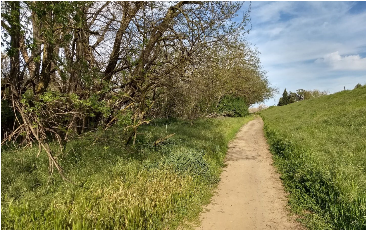
Photo 4: Facing east on Segment 4. The proposed trail would require vegetation removal at this location due to narrow width of existing track on levee toe.
