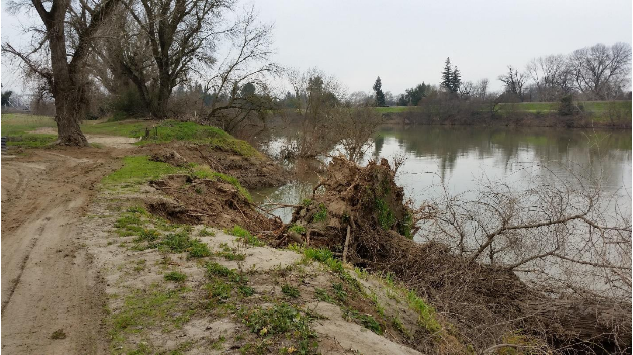
Figure 7. Example of Recent Bank Erosion and Limited Tree Cover Protecting Steep Erodible Banks on LAR at RM 6.0 Right Bank on Campus Commons Golf Course
