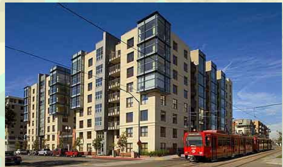
Unknown project 8-story residential San Diego, CA
