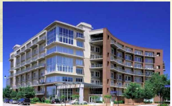
8-story residential RTKL, architects
