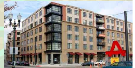
Sitka Apartments 6-story mixed use Portland, OR
