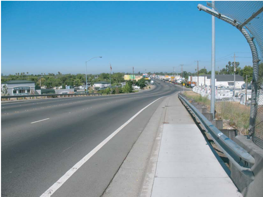
El Camino Avenue looking West from Railroad Track Overpass
