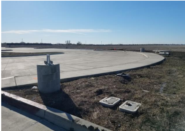
PHOTO 2.4-1: Partially Constructed Morrison Creek RT Station
