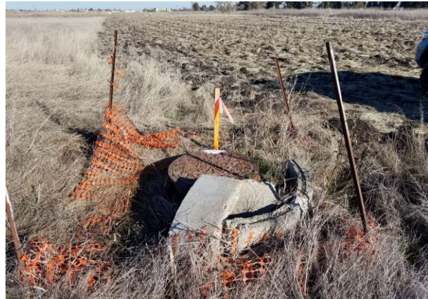
PHOTO 2.4-2: City of Sacramento Manhole Located Within Utility Easement
