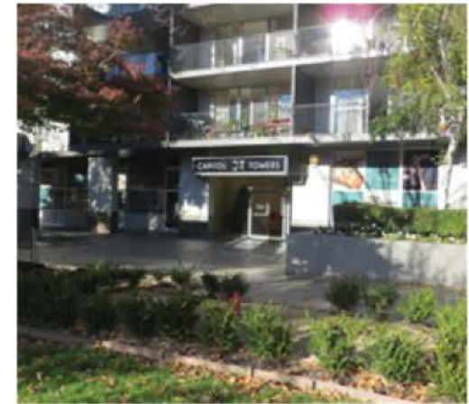
⑤ Capitol Towers Entry from Walks
