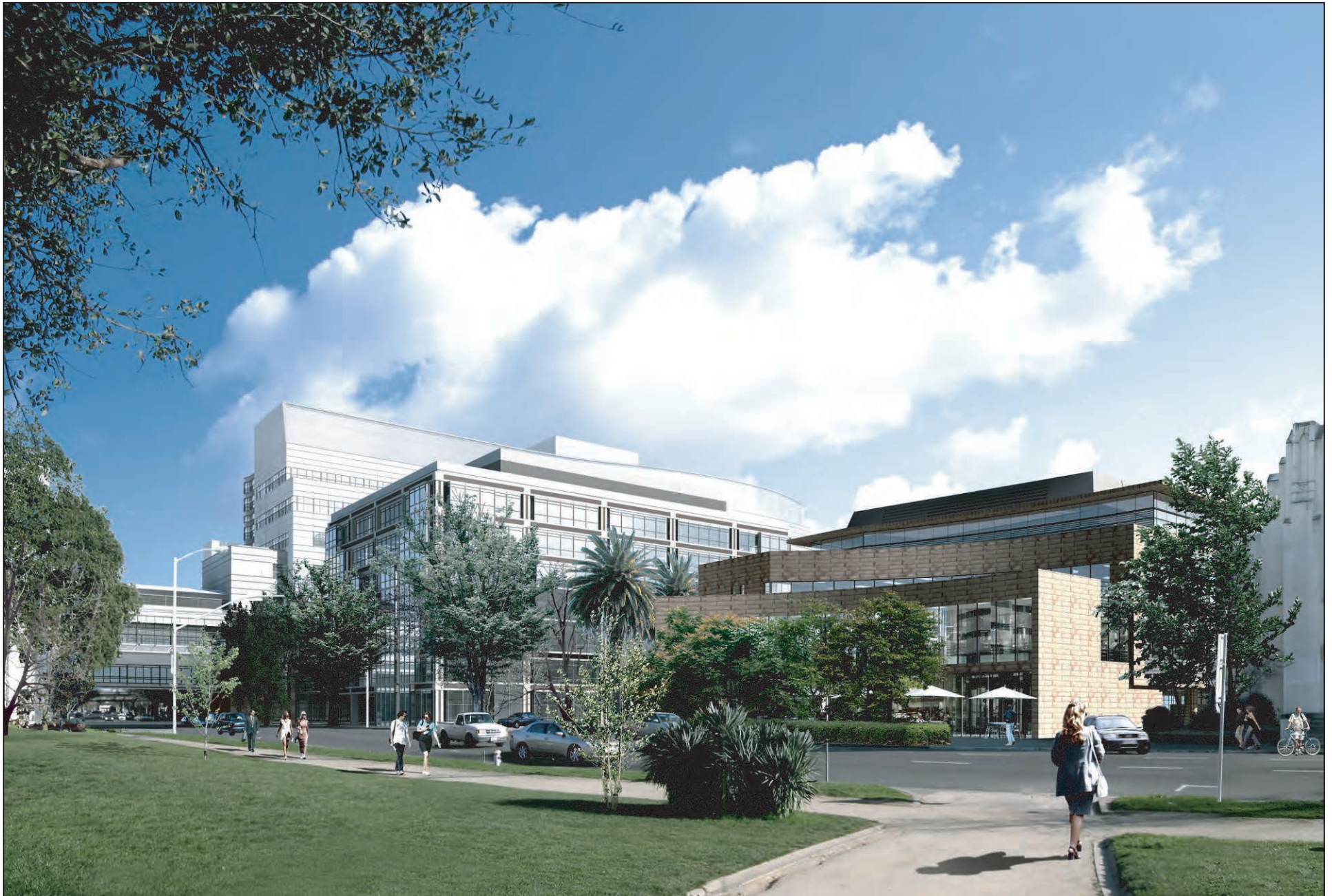
FIGURE 6.1-13 SMF Building, North Elevation
