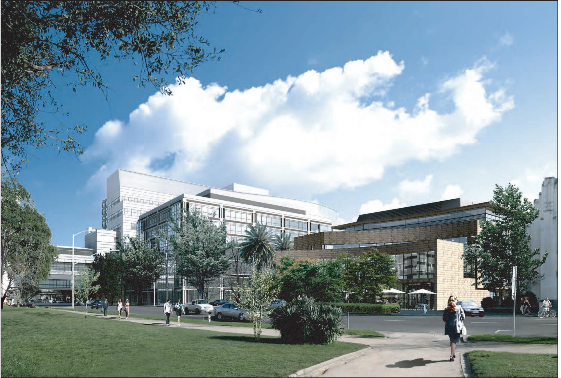
FIGURE 2-12 SMF Building, North Elevation
