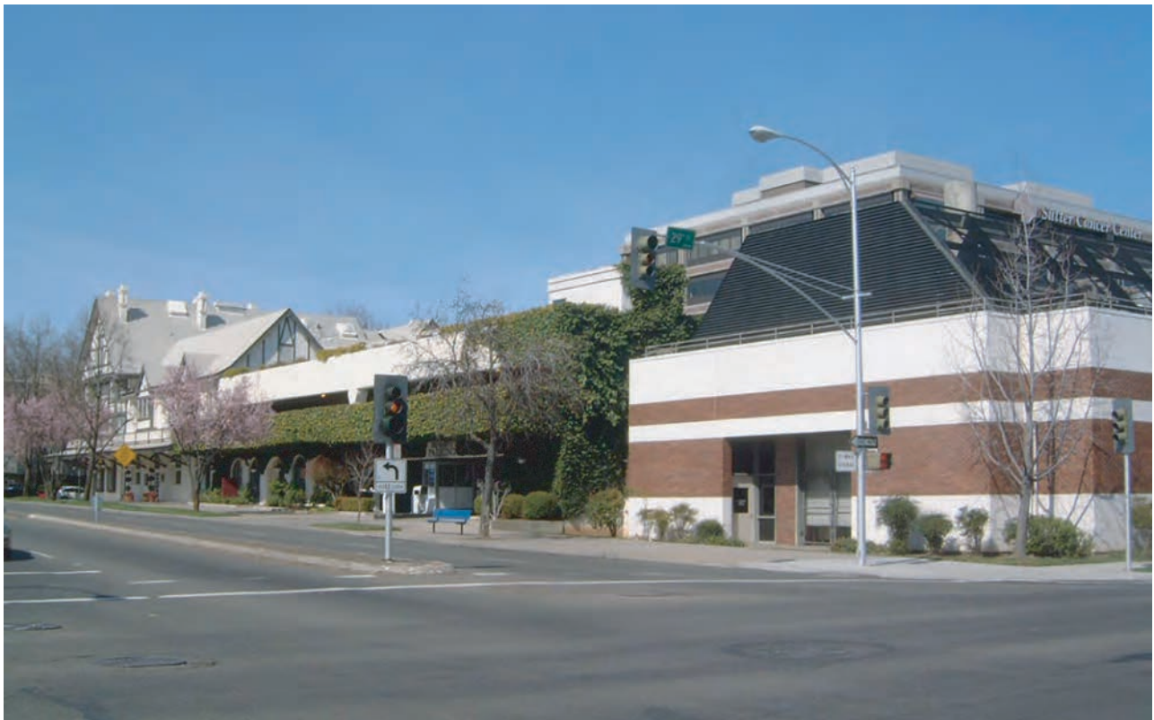
View 7: Sutter Energy Center, Old Tavern Parking Structure, (former) RAS Office, and Old Tavern from Capitol Avenue and 29th Street
