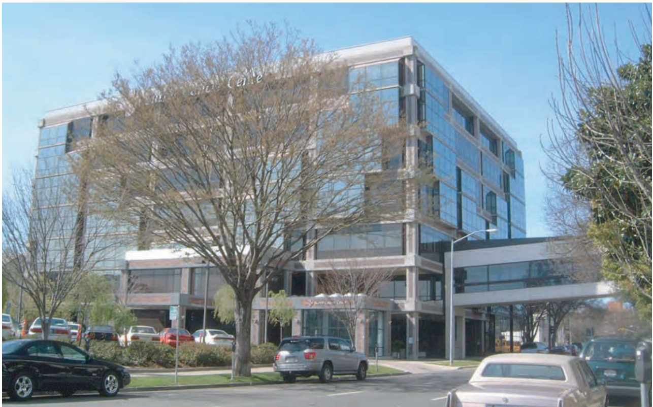
View 5: East side of Buhler Building on L Street
