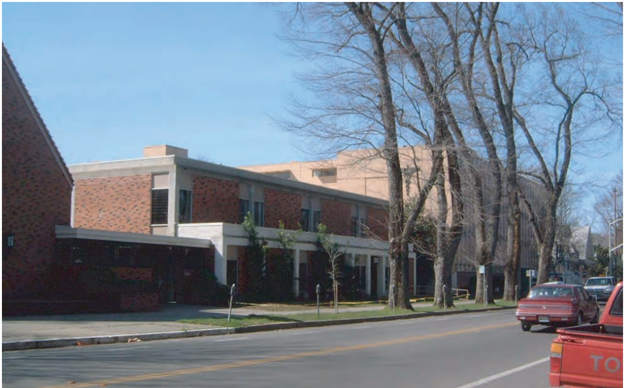
View 10: Trinity Cathedral Administrative Annex Building and St. Luke's Medical Office Building looking west on Capitol Avenue
