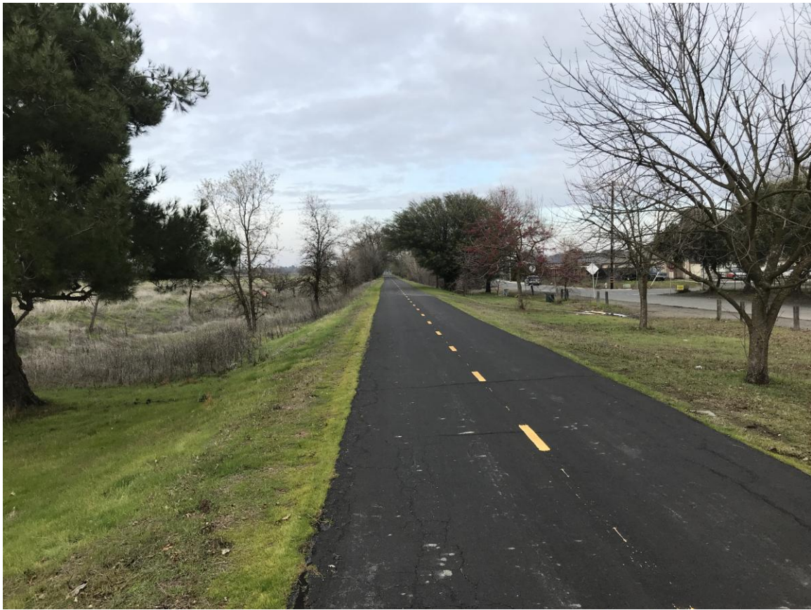
Bike path east of south end of Site from south to north.
