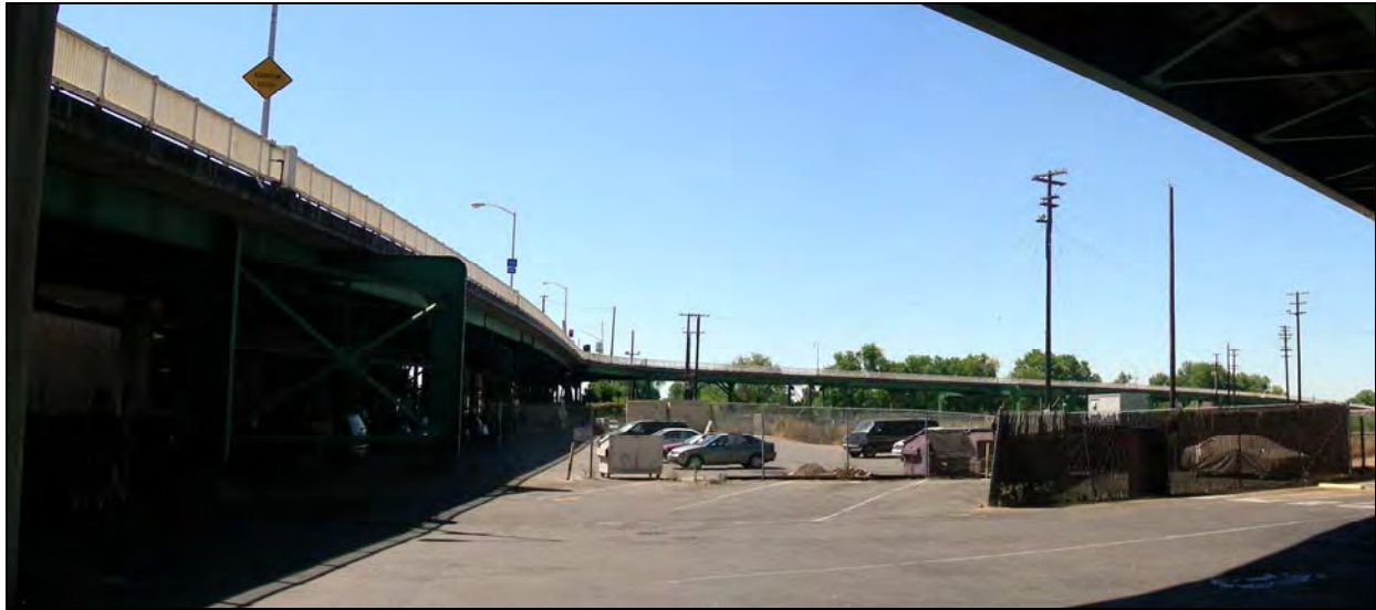
Photograph 13: I Street Bridge Eastern Approaches – I Street Viaduct and Jibboom Street Overhead, camera facing west, July 2007.
