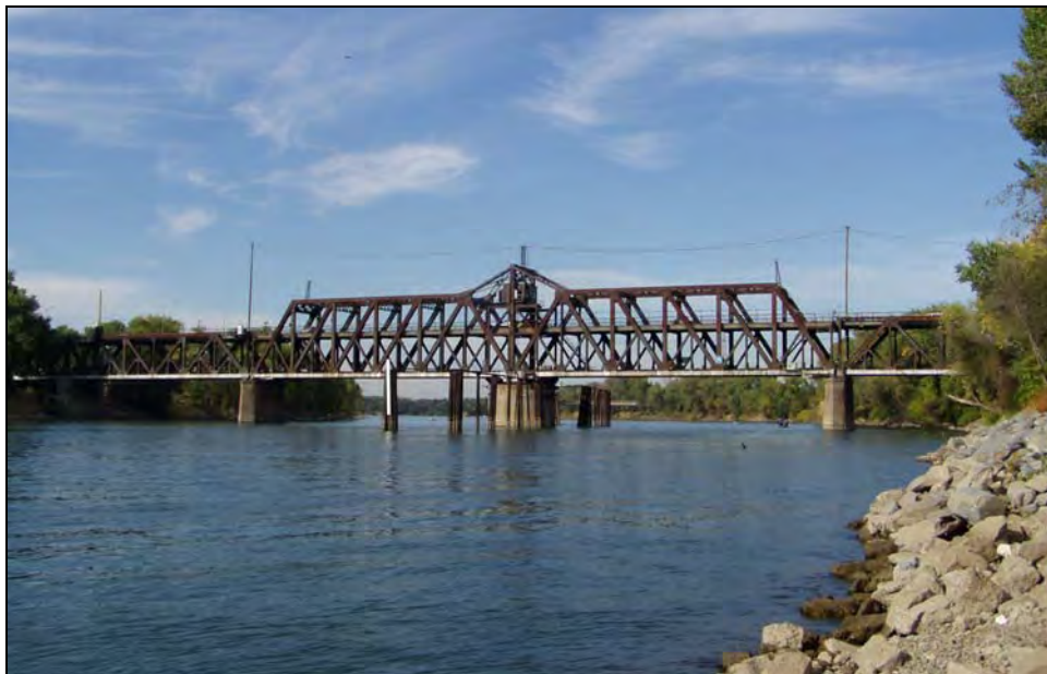
Photograph 12: I Street Bridge over Sacramento River, camera facing north, 2003.
