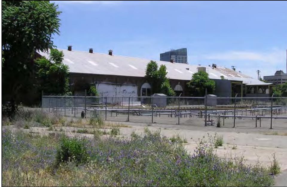
Photograph 6: Paint Shop, west side, camera facing southeast, June 2006.
