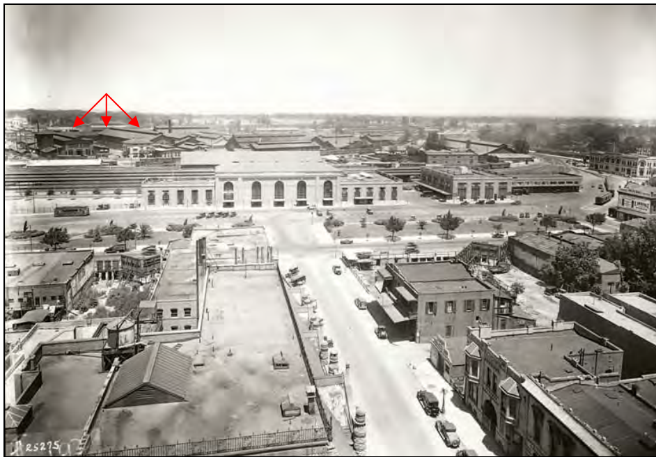
Photograph 16: Fourth Street, Sacramento Depot, and Southern Pacific Railyards, 1929. [Courtesy California State Library]. The red arrows indicate the location of extant buildings in the Central Shops District.
