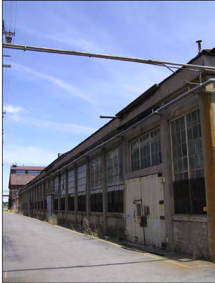
Photograph 5: Blacksmith Shop, west side, camera facing north, June 2006.
