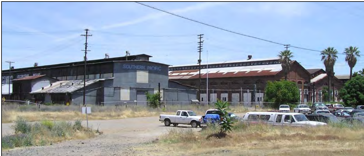
Photograph 9: Boiler House and Erecting Shop, camera facing northeast, June 2006.
