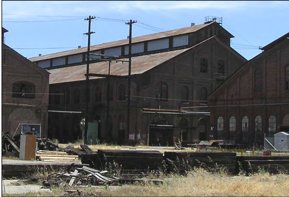
Photograph 2: Planing Mill, camera facing southeast, June 2006
