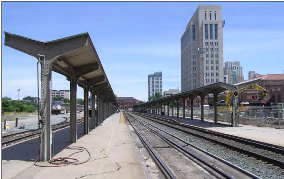
Photograph 11: Umbrella Sheds and Platforms, Sacramento Depot, camera facing east, June 2006.
