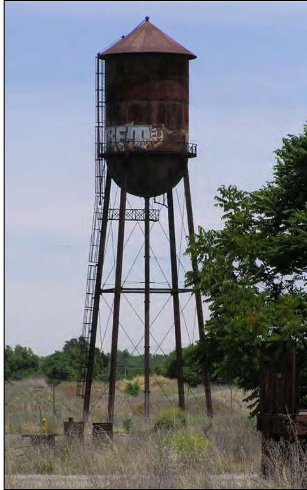
Photograph 8: Water Tower, camera facing north, June 2006.
