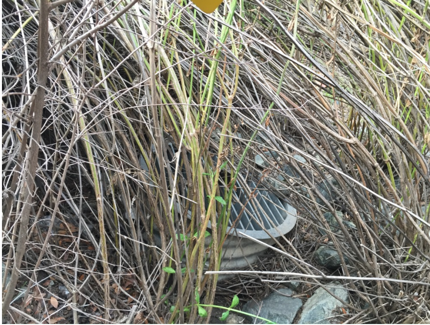
View of drainage intake within the feature during wet season (December 17, 2015)
