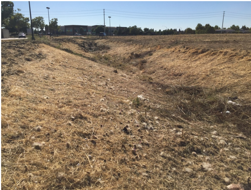
View of the feature facing west from within the project site during the dry season, following clearing of vegetation (July 27, 2016)
