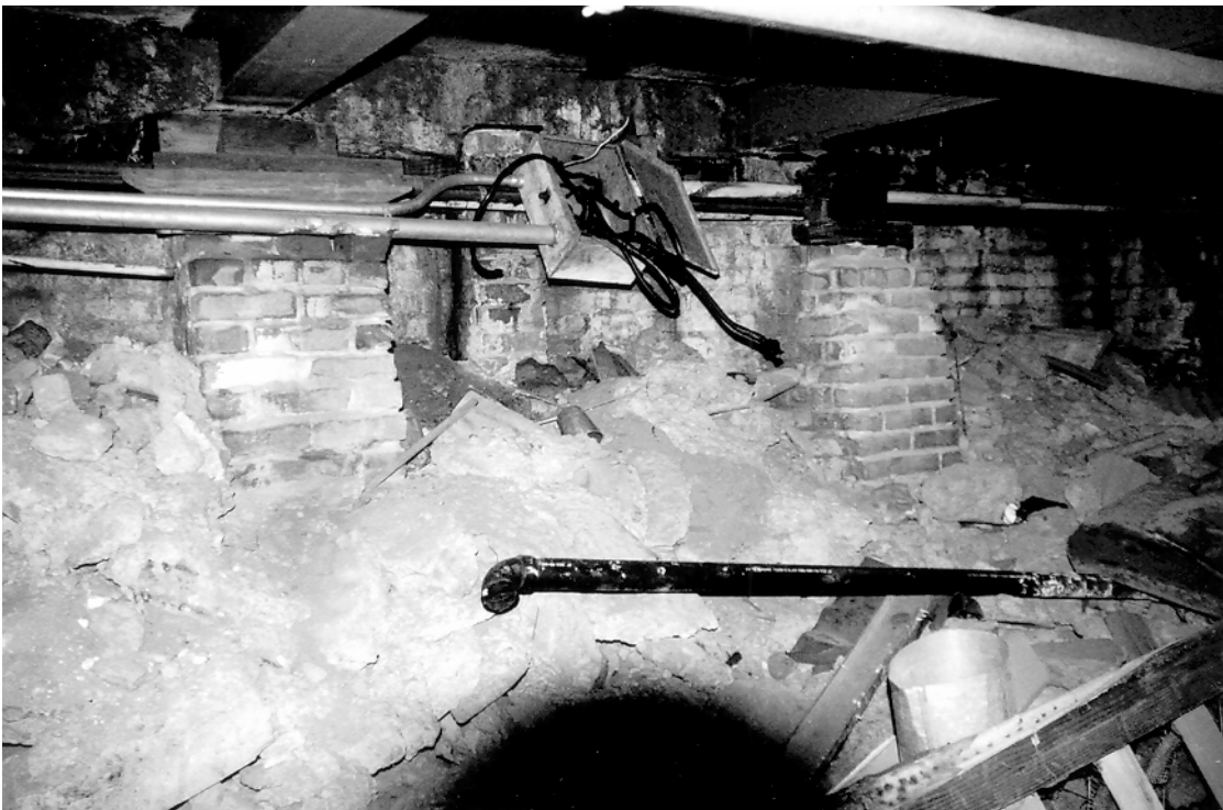
The Sacramento Underground beneath the sidewalks at The Broiler 1013-15 J Street.
