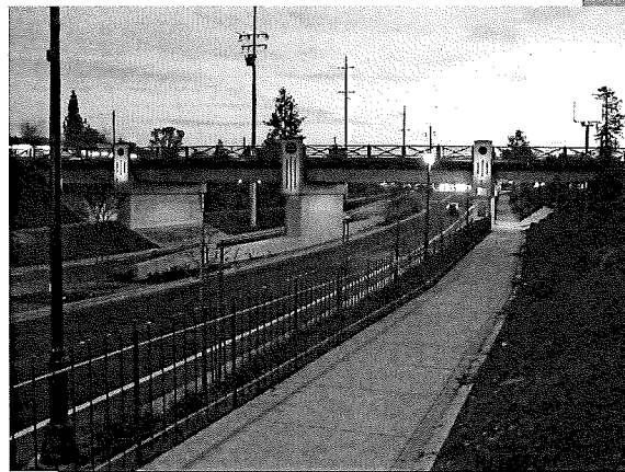
Completed Grade Separation At Night
