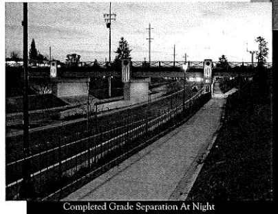
Completed Grade Separation At Night
