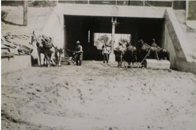
Beginning in 1912, Sacramento constructed its first underpass through the B St RR embankment. Further accesses were added over the years along with floodgates. With the addition of each new underpass or cut through the UPRR levee, the risk of flooding of
