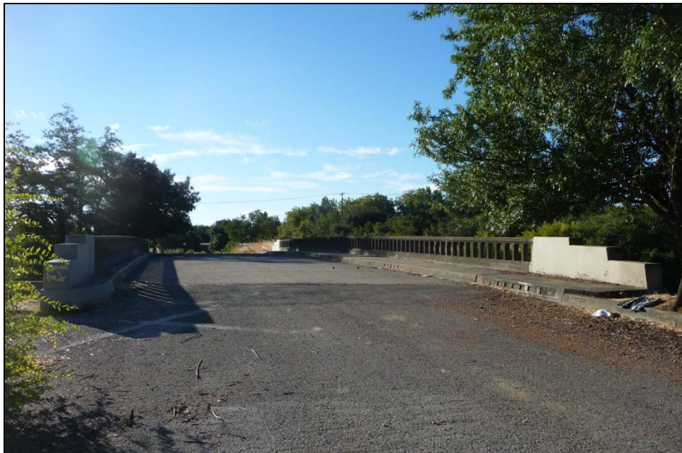
Photograph 1: A Street OC deck, camera facing east, 8/16/13.
