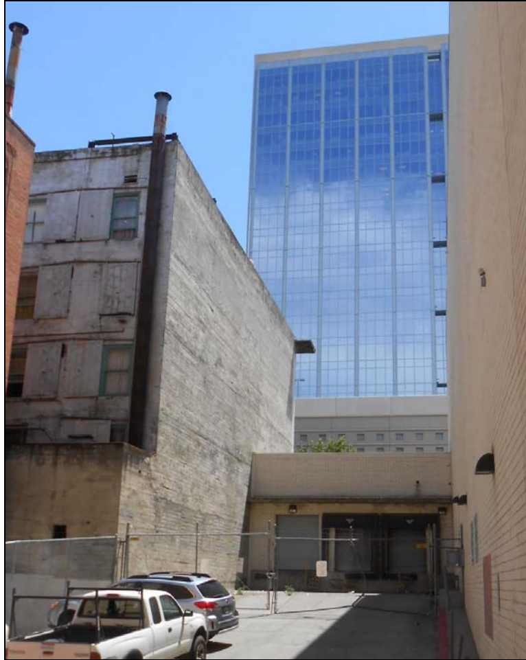
Photograph 3: View of Hotel Marshall west wall with projecting wrap-around cornice at site of proposed practice facility, camera facing south, July 16, 2014 (ESA).
