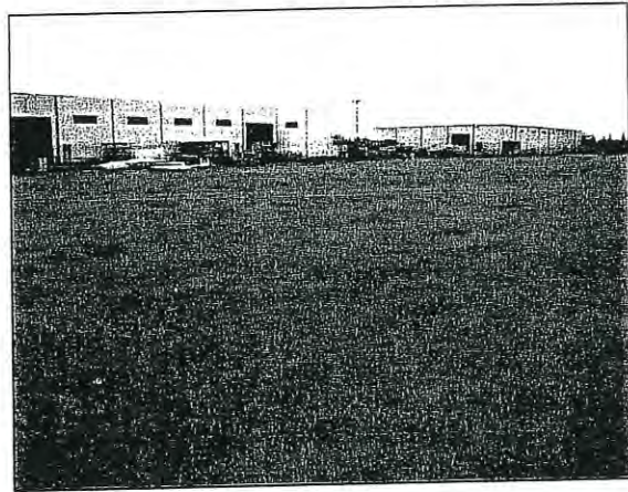
View of commercial land use southeast of project site.
