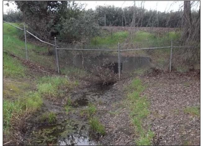
**PHOTO 2:** Existing 3' x 4' box culvert (January, 2015).
