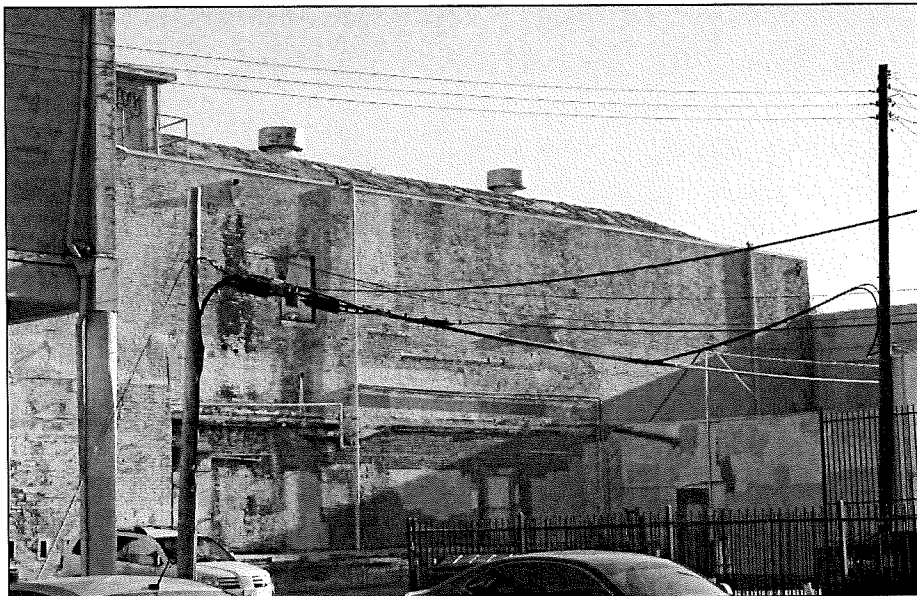
Photograph 9: South side of Building 2, camera facing northeast, February 27, 2015.
