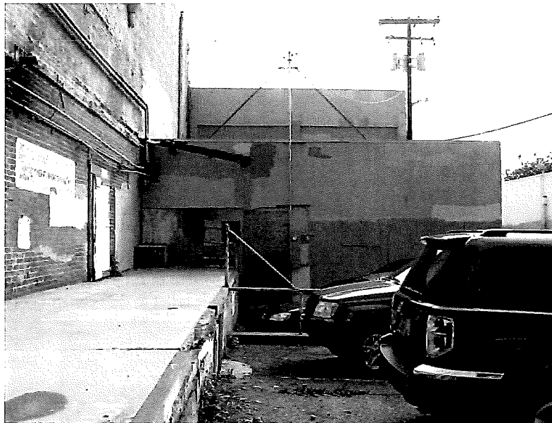
View east of Section 5, with Section 3 loading dock to left (Accession 08-8007-DIG-1-29, Feb. 24, 2009)
