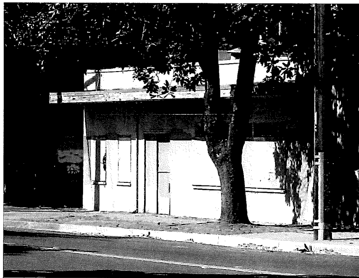
View southwest of one-story office addition fronting on 17th Street. Accession 08-8007-DIG 2-025, 04/05/09
