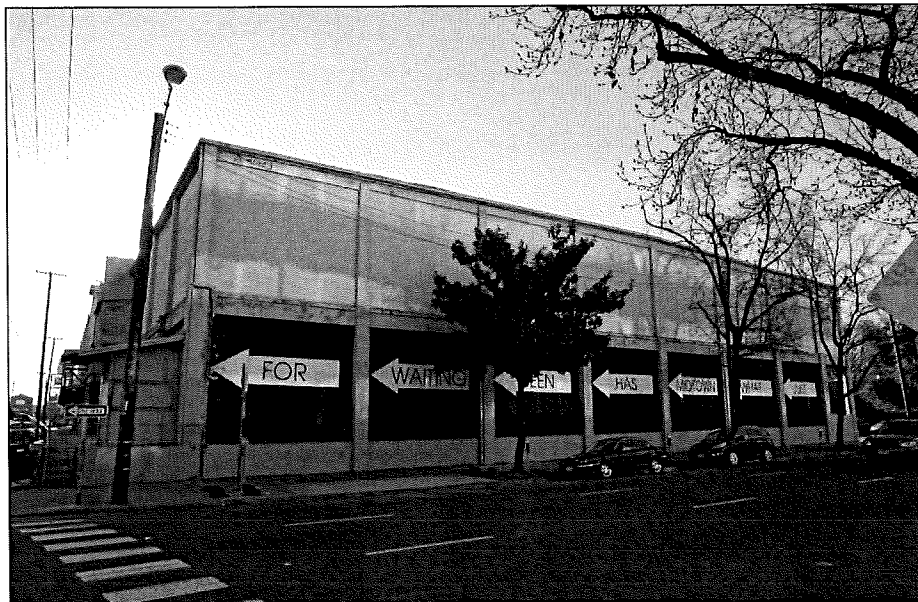
Photograph 6: West side of Building 1, camera facing east, February 27, 2015.
