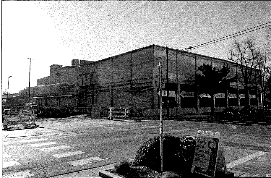
Photograph 1: Crystal Ice and Cold Storage property, north and west sides along R and 16 th streets, camera facing southeast, February 27, 2015.
