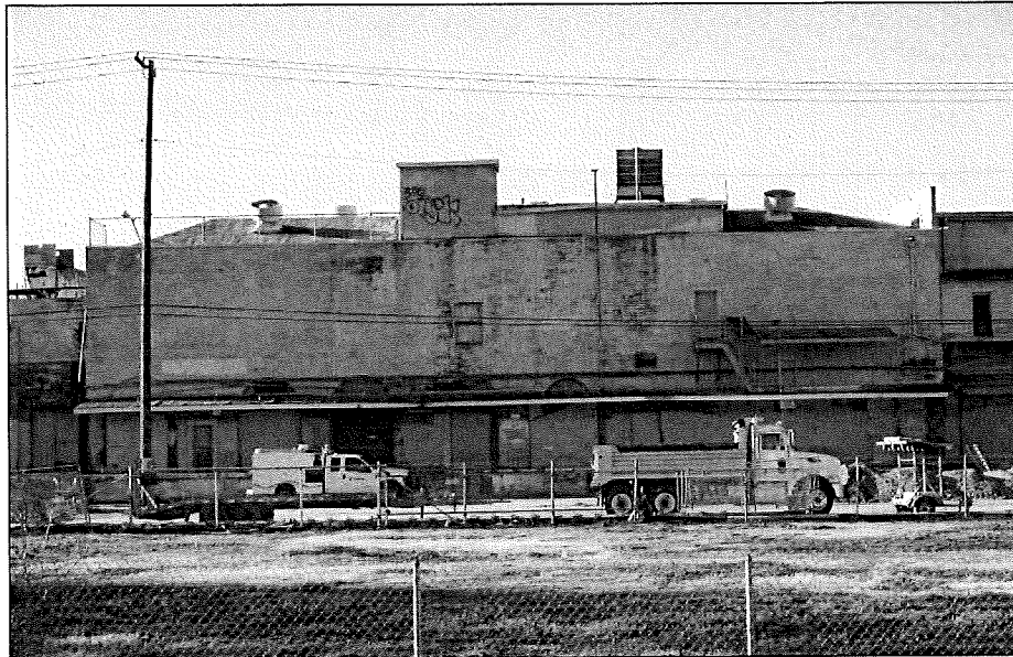
Photograph 7: North side of Building 2, camera facing southeast, February 27, 2015.
