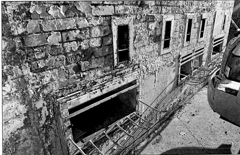
Photograph 8: Detail view of ice dispensers, camera facing northeast, February 27, 2015
