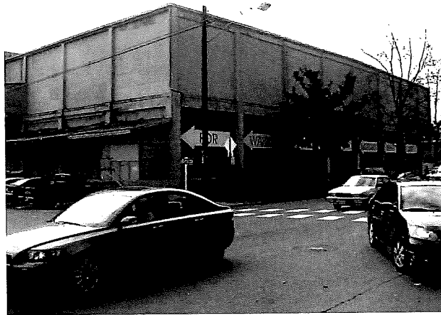
View southeast of north and west façades, Section 4 (Accession 08-8007-DIG-1-003, Feb. 24, 2009)
