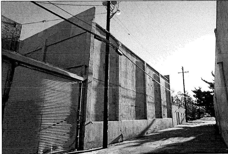
Photograph 11: South side of Building 3 Truck Storage addition, camera facing northeast, February 27, 2015
