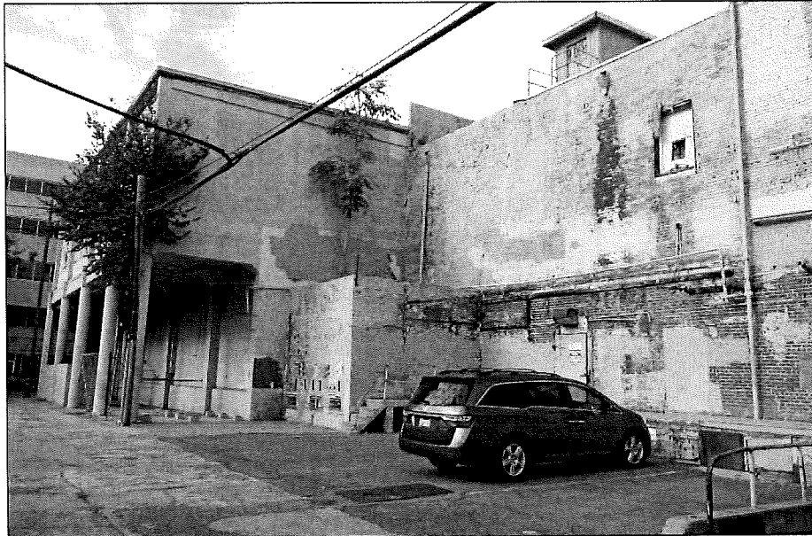
Photograph 10: Ice Chute located at alley (left), camera facing northwest, October 30, 2014
