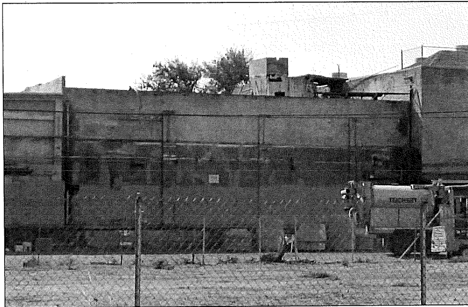
Photograph 10: North side of Building 3, camera facing south, October 30, 2014.
