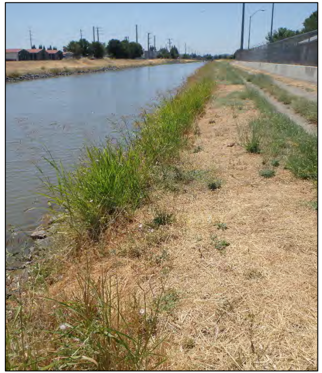
Photo 6. Drainage canal located at Well 39.
