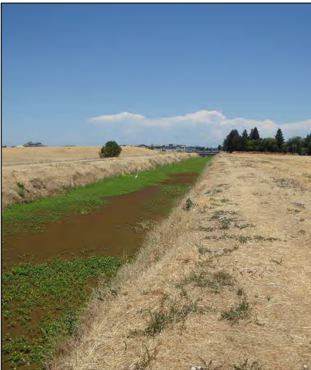
Photo 7. Drainage canal located at Well 15.
