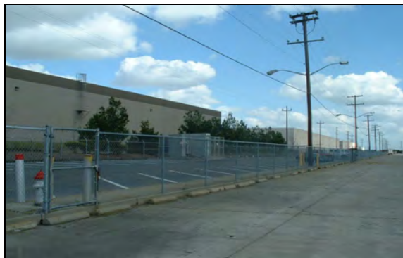
Photo 20 – Northern adjacent warehouse/light industrial buildings
