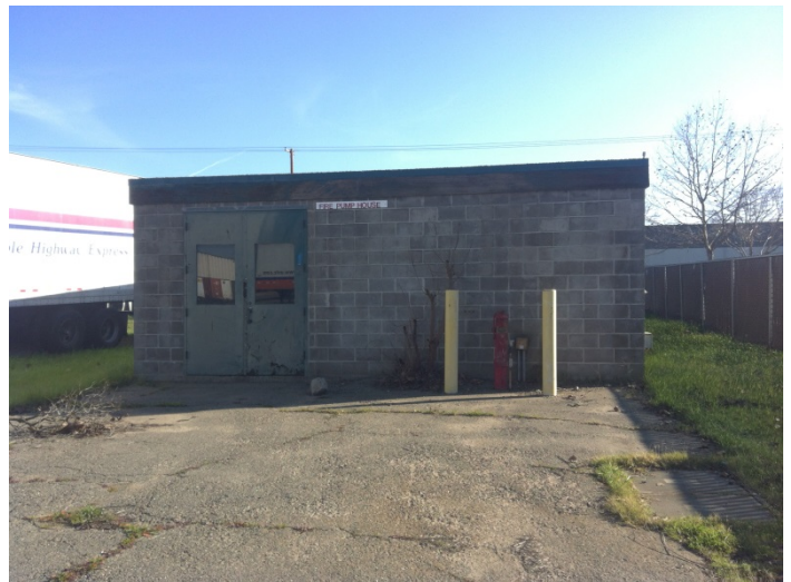
20. View of the west side of the fire pump house located in the southeast corner of the subject property
