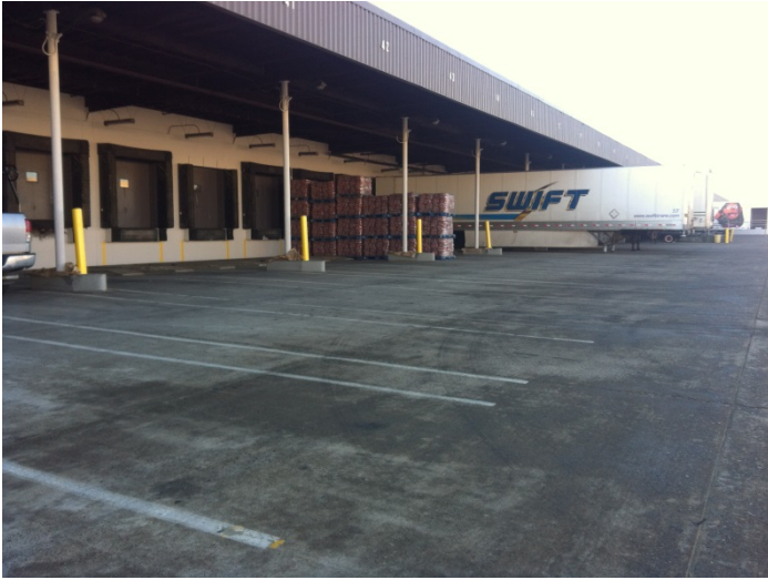
13. View of a typical truck loading dock area along the north side of the main subject property building
