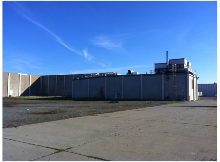
32. View of the southwest side of the main subject property building from the west
