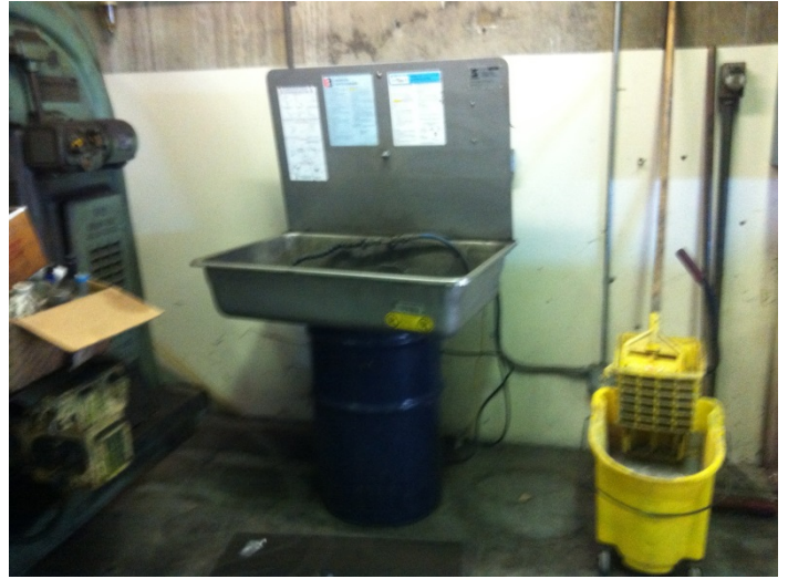
38. View of an aqueous parts washer in the maintenance area
