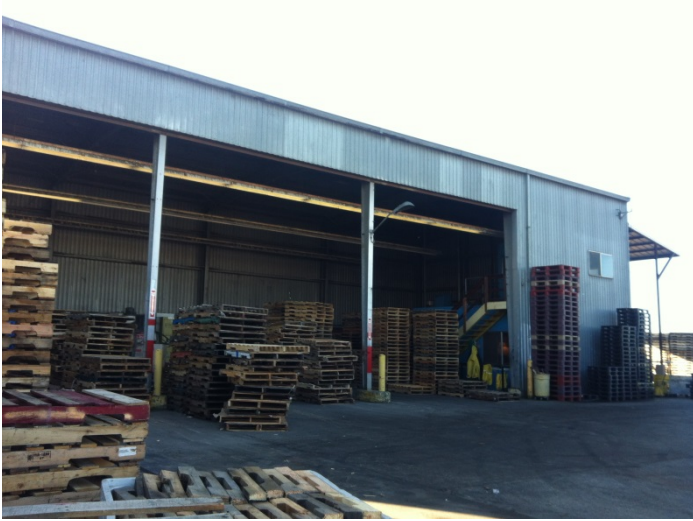
25. View of the north side of the metal storage structure from the northeast
