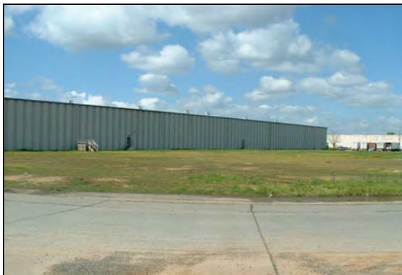
Photo 3 – Subject building from the southeast
