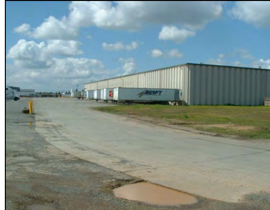
Photo 2 – Subject building from the southeast
