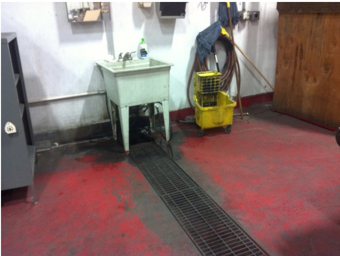
43. View of a sink leading to a system of trench drains throughout the main subject property building which ultimately lead to the sewer system
