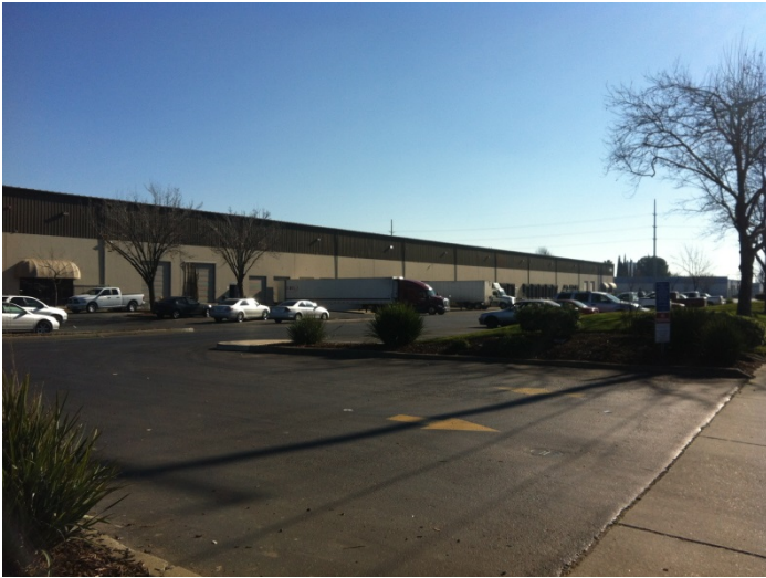
59. View of the east adjacent commercial/industrial building from the northwest
