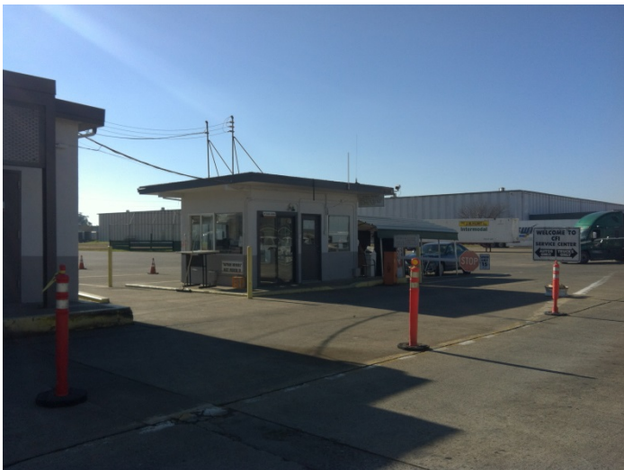
3. View of the northeast side of the guard booth on the northeast side of the subject property, from the northeast
