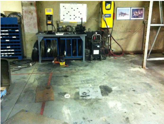
39. View of staining observed in the maintenance area
