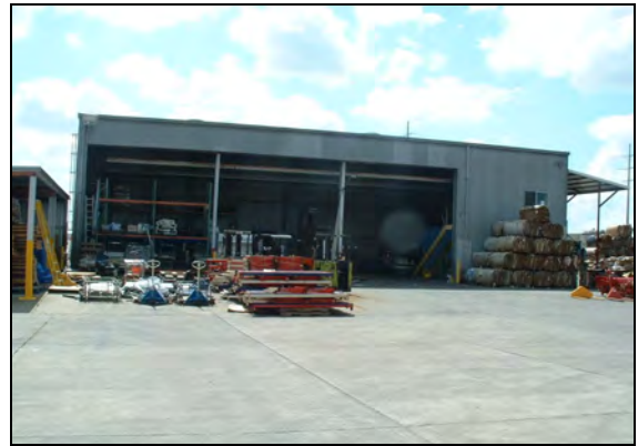
Photo 14 – The shed south of the warehouse
