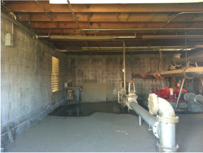
21. Interior view of the fire pump house
