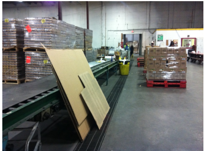
44. View of one of several trench drains throughout the main subject property building
