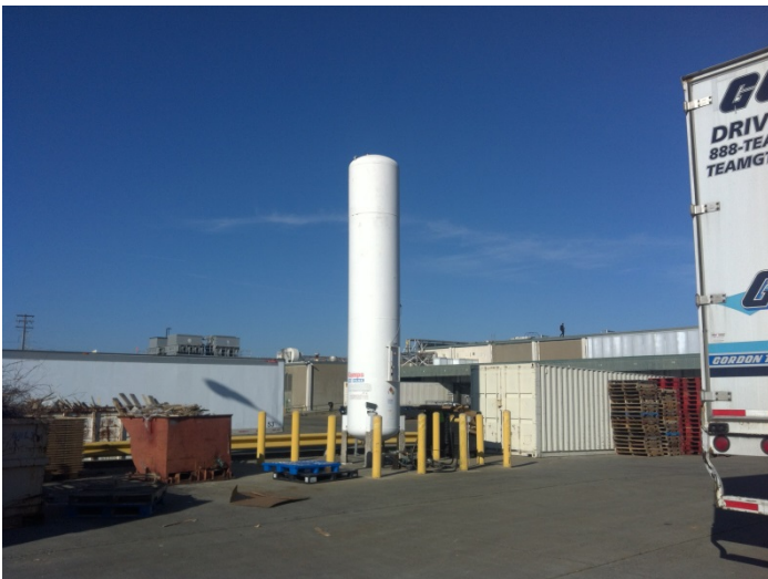
23. View of the propane AST located near the southwest corner of the site
