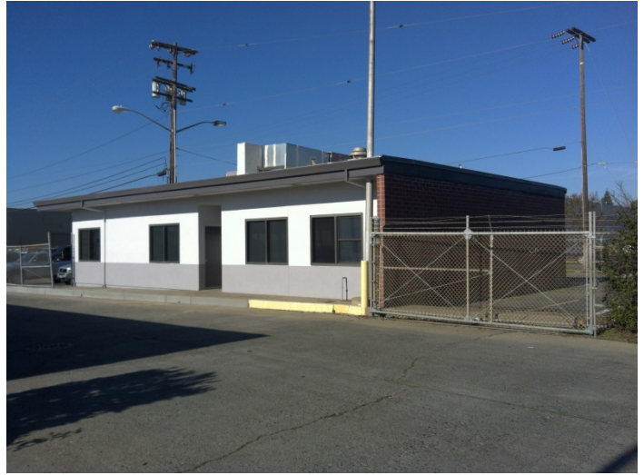
2. View of the southeast corner of one of two office structures on the northeast side of the subject property, from the southeast
