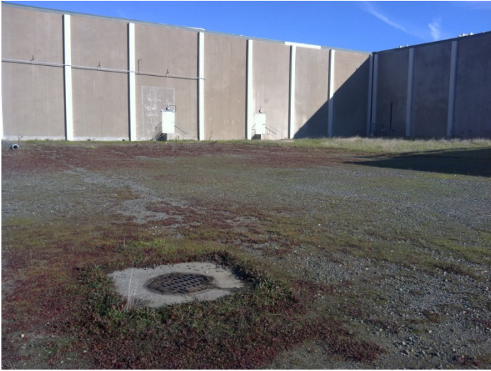
33. View of a storm drain located south of the westernmost portion of the main subject property building
