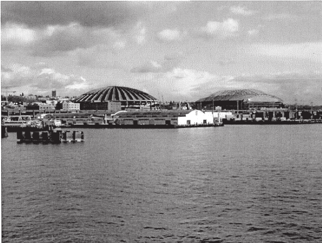
The Kingdome and its replacement, Safeco Field ("built to resemble the great ballparks of yesteryear 2 "), Seattle, WA. March 2000. Photo by Charlene Roise.
