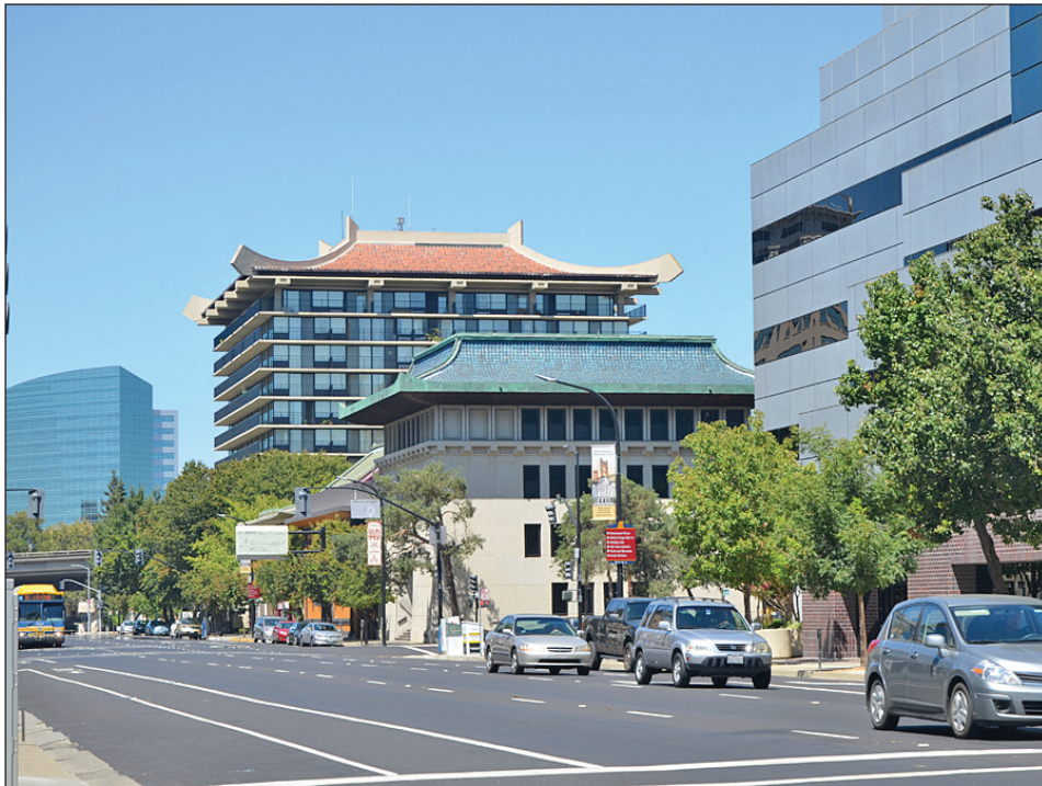
PHOTOGRAPH 5. Looking north across J Street at the Ping Yuen Building and Wong Center from 6th Street and J Street intersection.
