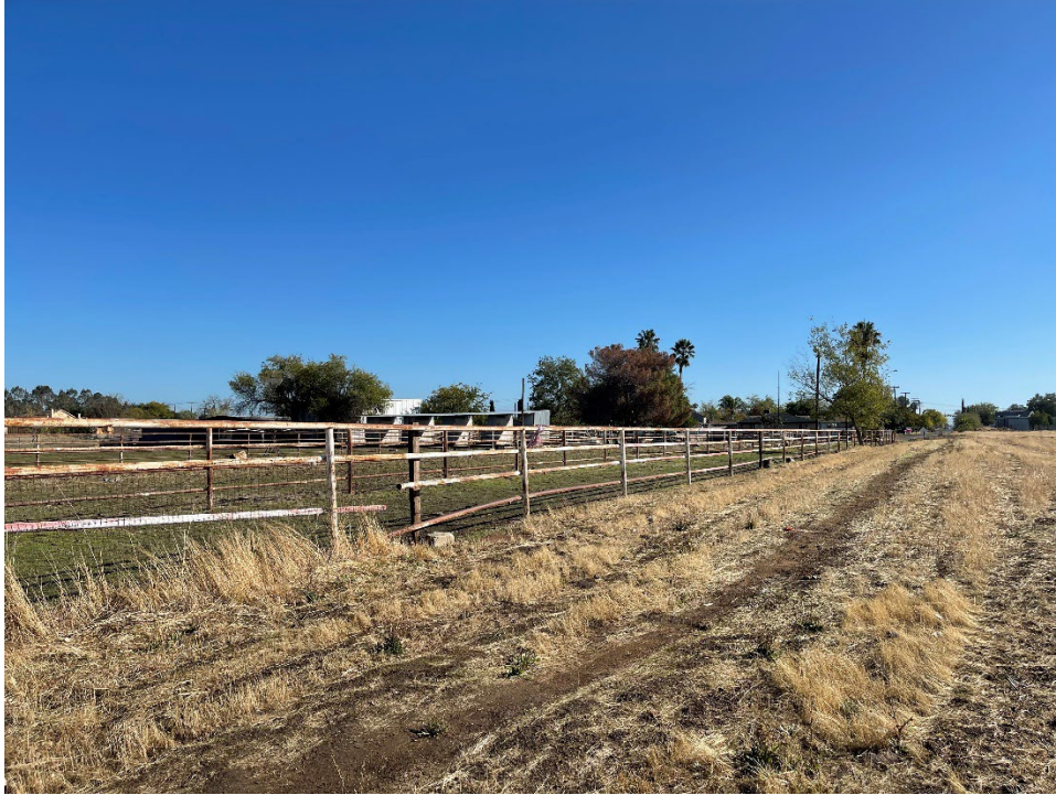
Photo 3. Photograph of the future construction site of Main Avenue, which will expand the existing Main Avenue west to Rio Linda Boulevard, north of the proposed residential community. Taken facing northeast (Oct. 2021).
