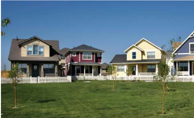
Homes should be designed to create variety in scale and architectural form/massing.
