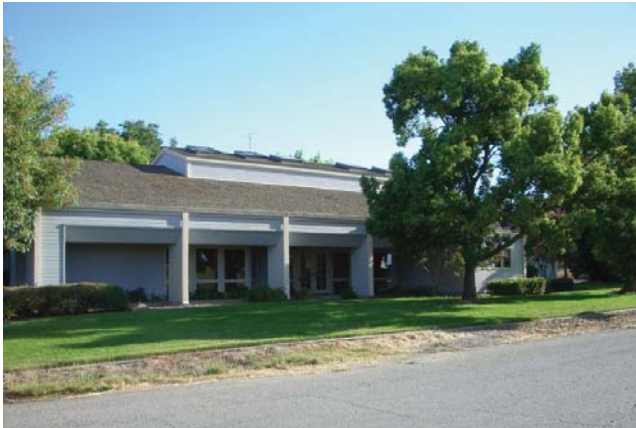
The Freeport community lacks curb gutters and sidewalks.
