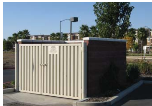
A concrete apron in front of the trash enclosure facilitates pickup and protects adjacent asphalt.
