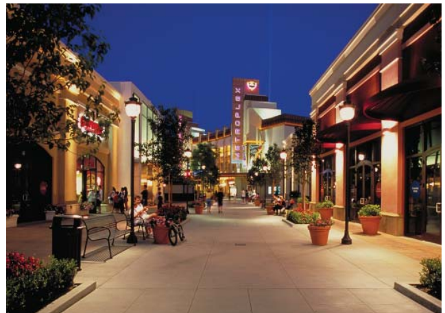
Buildings at the ends of the Village Center Plaza can serve as landmarks that anchor the plaza by incorporating corner and entry features that exceed the height of the building.
