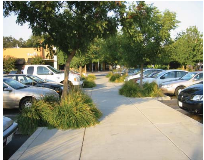
Major pedestrian access and routes through parking lots should be clearly defined with change in color and material of paving.
