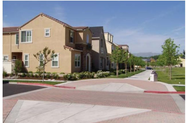
Wheelchair accessible sidewalks
