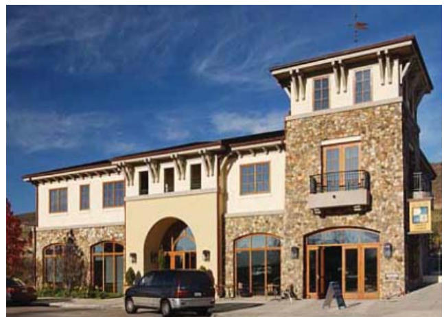
Building façades provide the interface between the built environment and the public realm.
