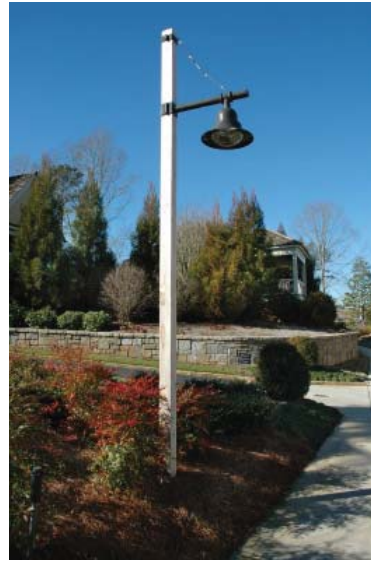
Landscaping around site lighting fixtures
