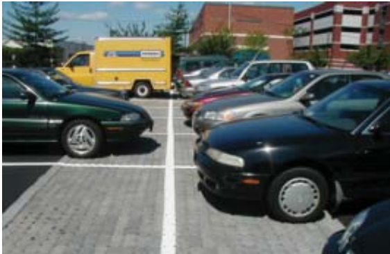
Permeable asphalt and concrete paving may be used in parking areas.
