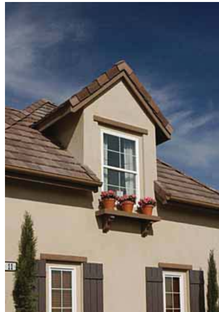
Dormer roof consistent with roof slope
