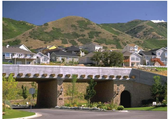
Bicycle and pedestrian bridge.
