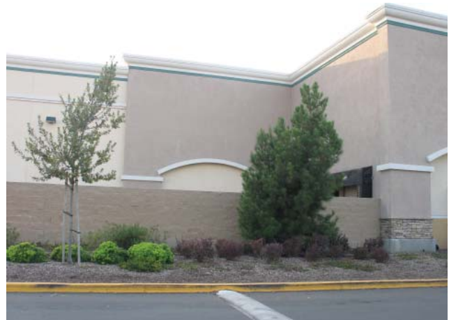
Loading areas should be placed unobtrusively at the rear side of the building and screened from view.
