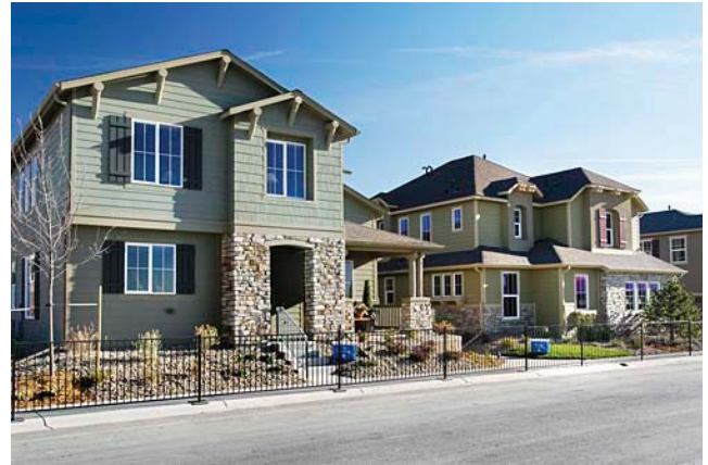
Lighter materials placed above stone base
