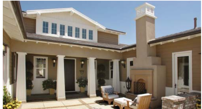
Ground floors of all homes should have an outdoor living space.
