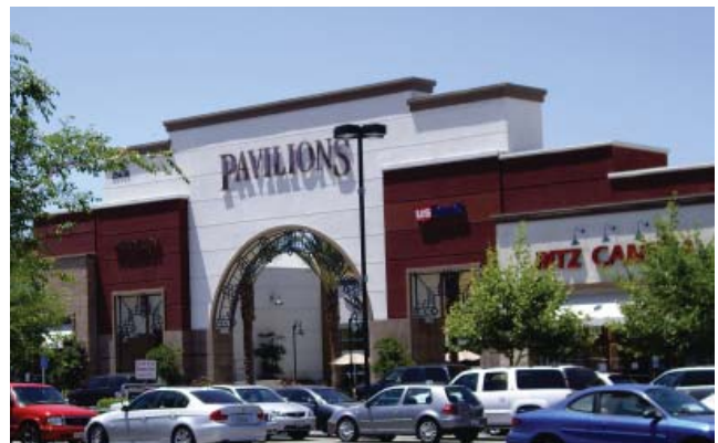
Variation of scale and massing help in maintaining human scale in the large format stores.
