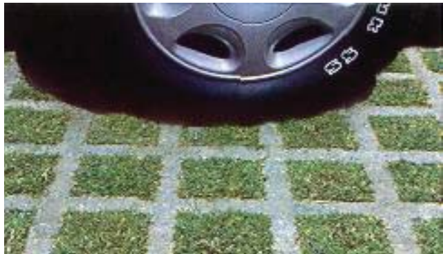
Visual appeal should be balanced with functionality through the selection of materials that allow stormwater runoff to stay on-site and contribute to groundwater recharge.
