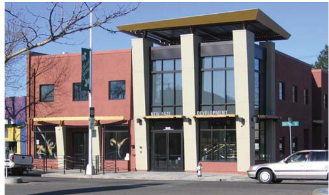
Contemporary canopies, awnings, and overhangs may be used over display windows and entryways to articulate the building facade.
