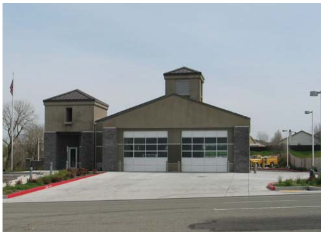
Site for a fire-station will be included within the Delta Shores Plan.
