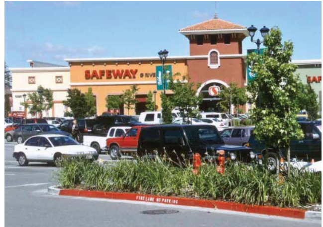
Trees planted in surface parking lots should be protected with curbs or tree grates, or located in landscaped walkways.
