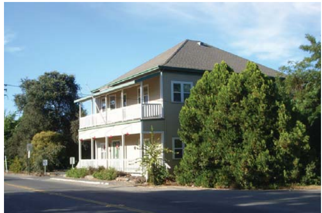
Typical porches and balconies on Freeport Boulevard.
