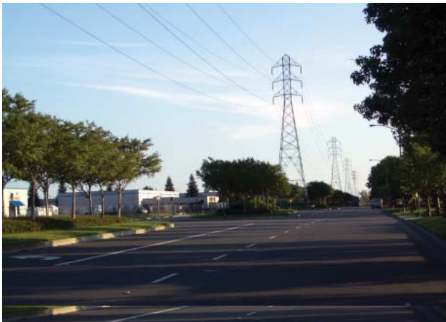
Typical photograph of electric towers within median.
