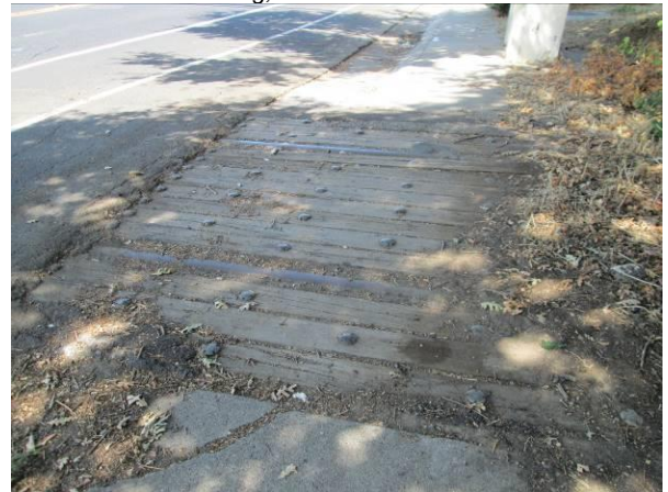
Image 14: Detail view of what appear to be wood overcrossing remnants at the 43 rd Avenue crossing.
