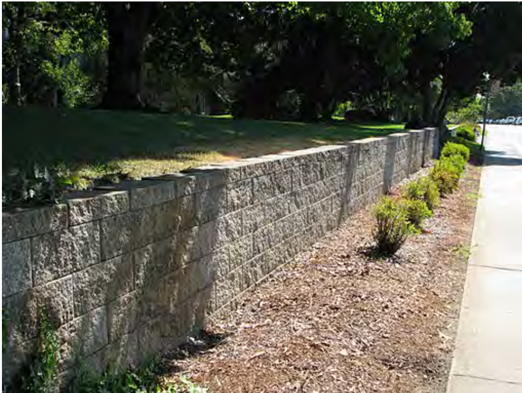
PHOTOGRAPH 62: New concrete block retaining wall along S Street.
