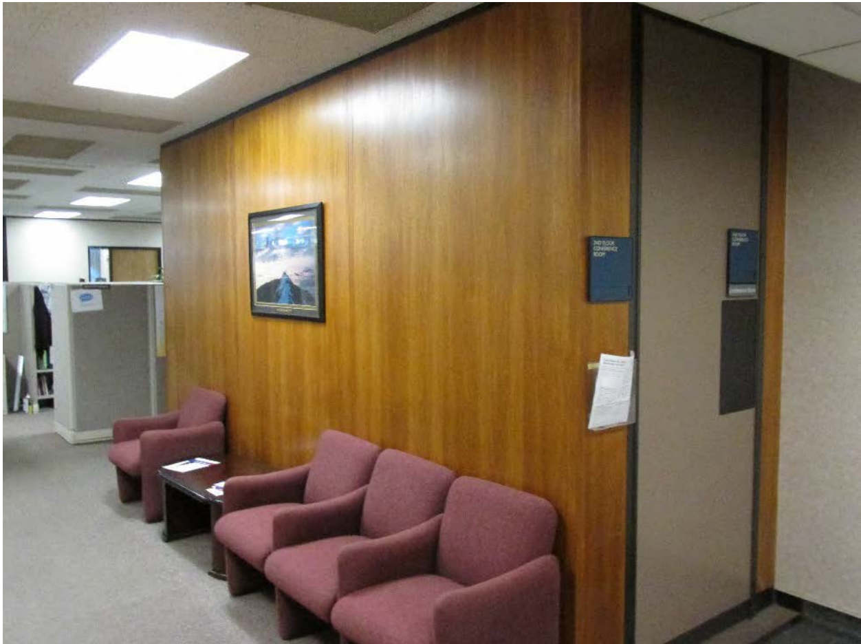
Figure 24. Typical original wood partitions.
