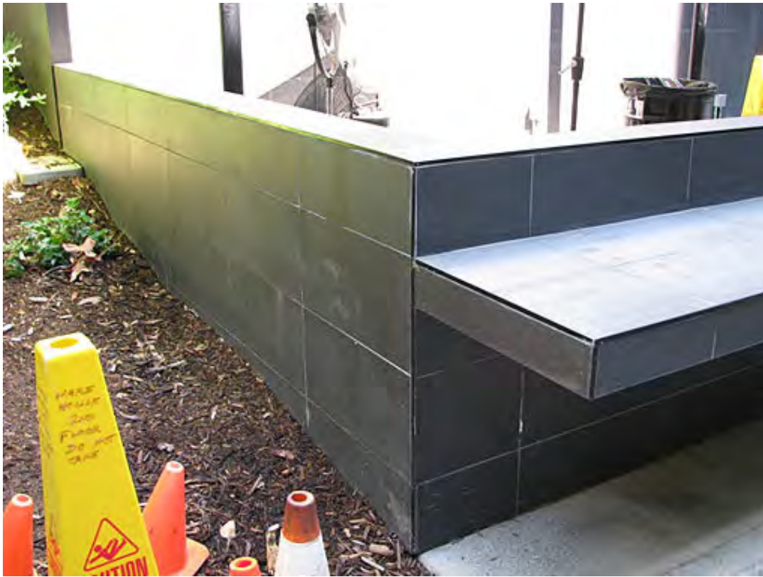
PHOTOGRAPH 71: Wall cladding at cafeteria terrace.
