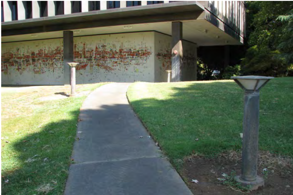
Figure 25. A 4-foot-wide, exposed aggregate concrete path that postdates initial construction.
