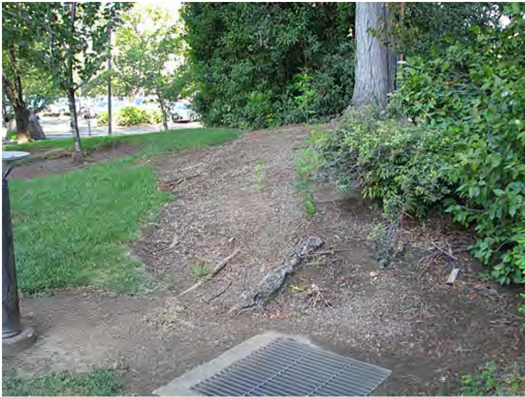
PHOTOGRAPH 29: Planting bed on a berm.
