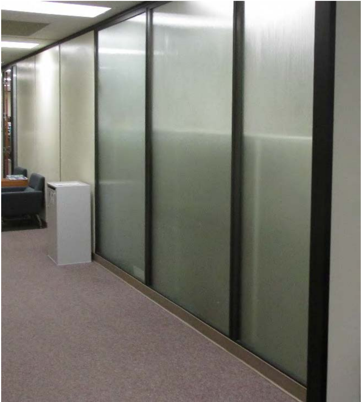
Figure 28. Typical original translucent panels.
