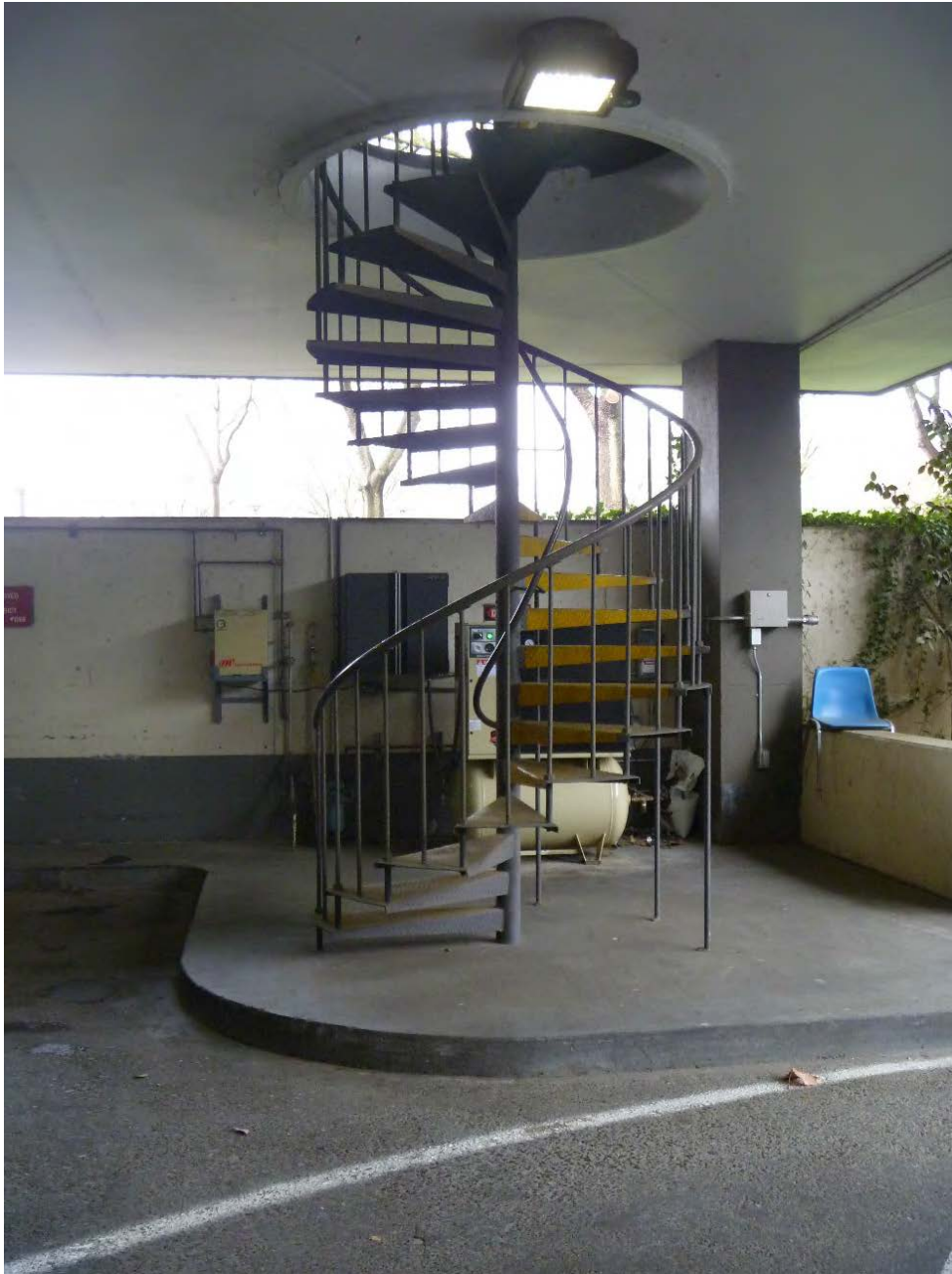
Figure 31. Parking garage staircase.
