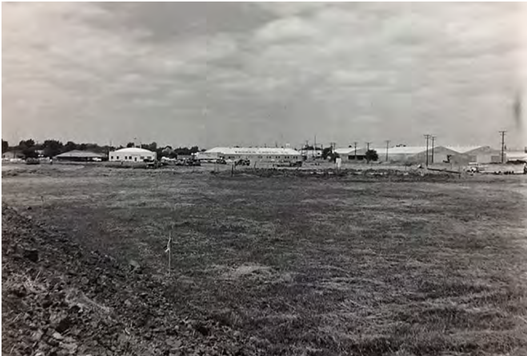
PHOTOGRAPH 1: May 12, 1958 photograph showing flat construction site at the location of the future headquarters building.
