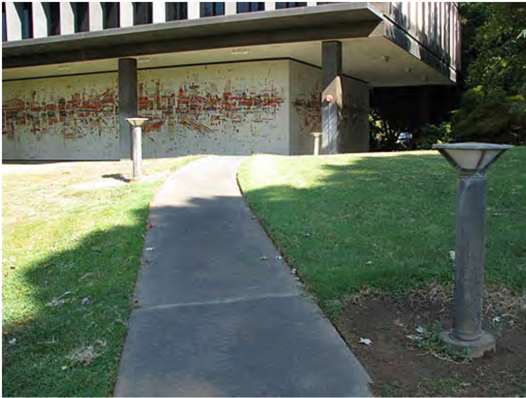
PHOTOGRAPH 19: Path to loggia. The path post-dates the original landscape construction.
