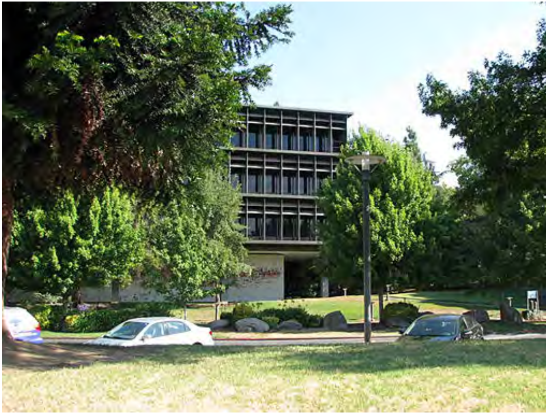
PHOTOGRAPH 12: Current view of the building from S Street.
