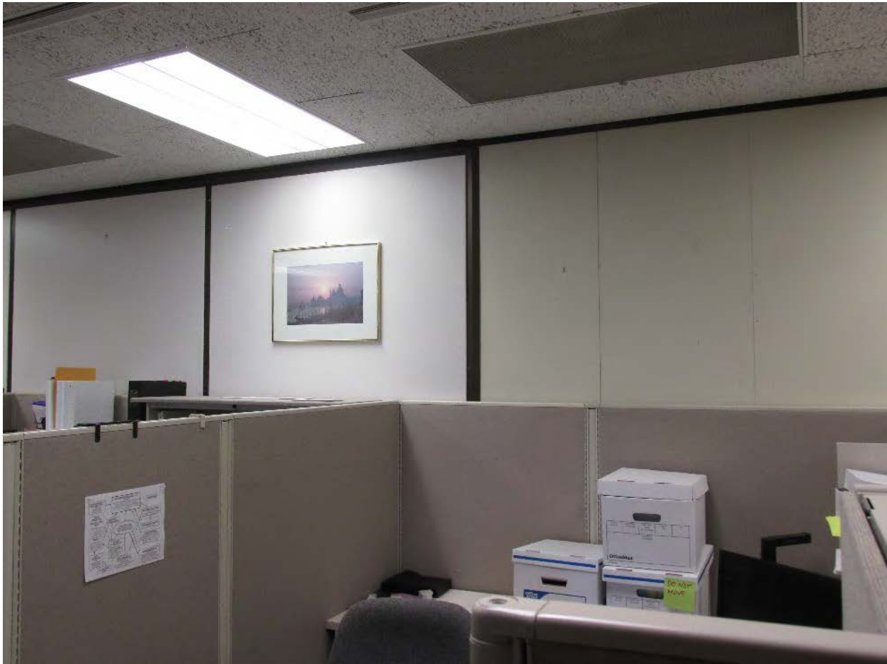
Figure 25. Typical original (left) and nonoriginal (right) vinyl partitions.
