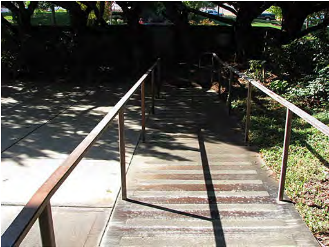
PHOTOGRAPH 25: Ramp with handrails at the entrance plaza.
