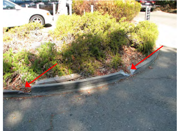
Figure 38. Broken curbs.
