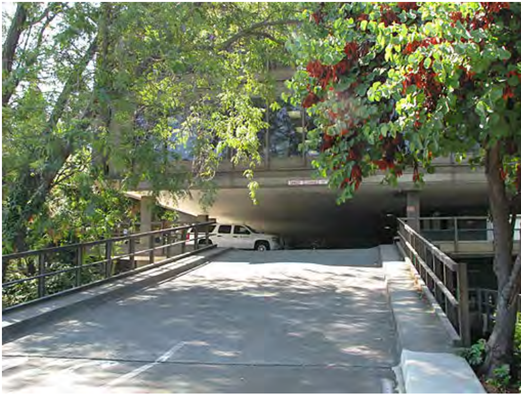
PHOTOGRAPH 53: Ramp to the structured parking.
