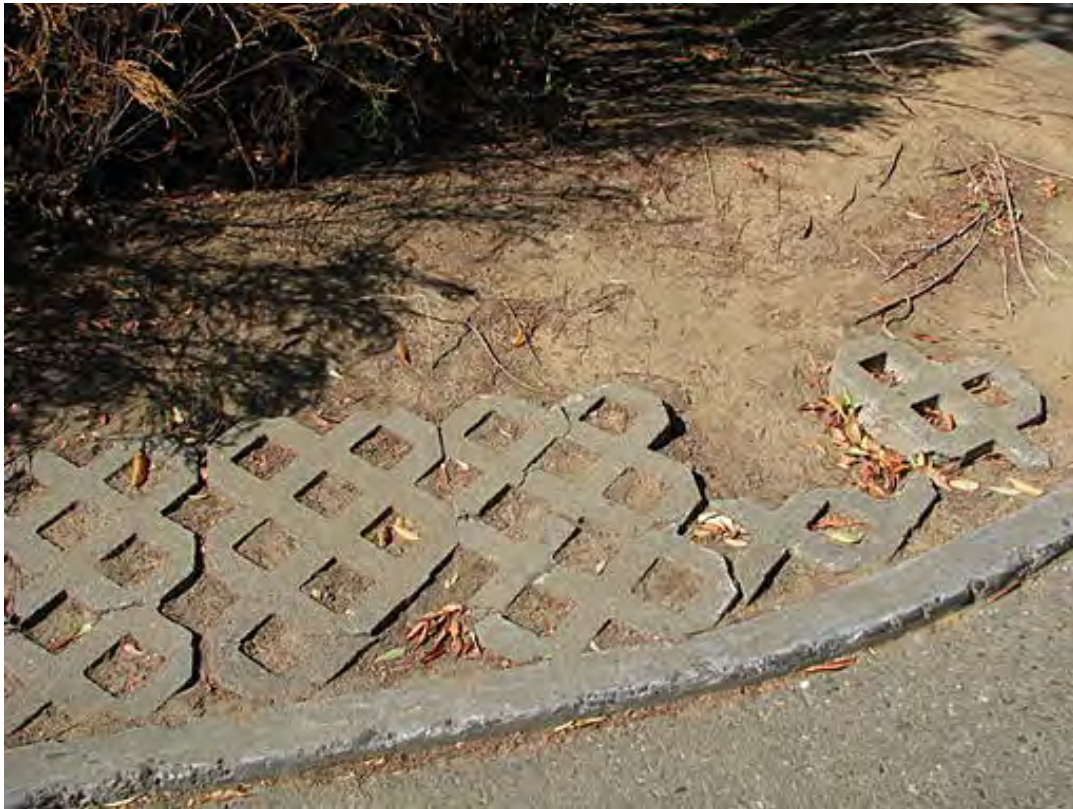
PHOTOGRAPH 40: New structural paving support for vehicles.
