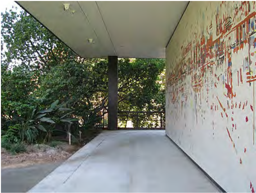
PHOTOGRAPH 27: View along the loggia.
