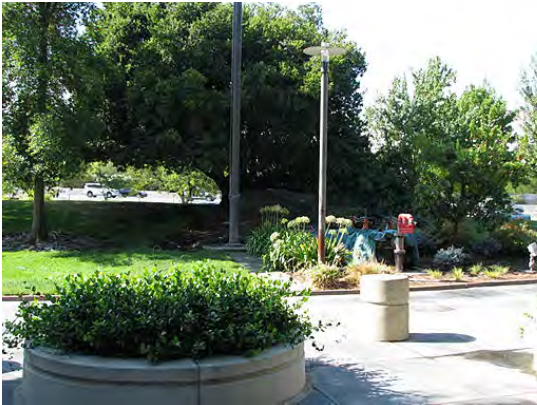
PHOTOGRAPH 5: New flagpole, planters, bollard, and mechanical equipment at the entry parking.
