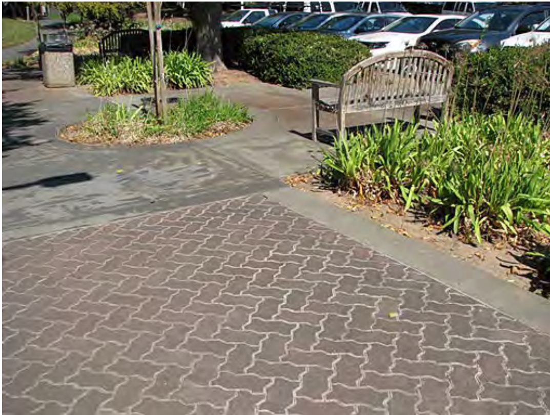
PHOTOGRAPH 60: Paving and site furnishings at the eastern parking area.
