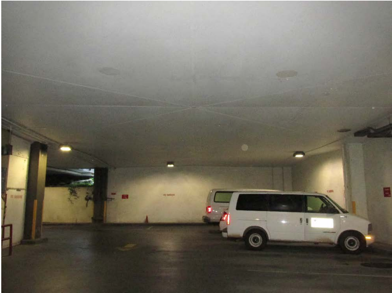
Figure 32. Underside of structural slab, lower level of parking garage.
