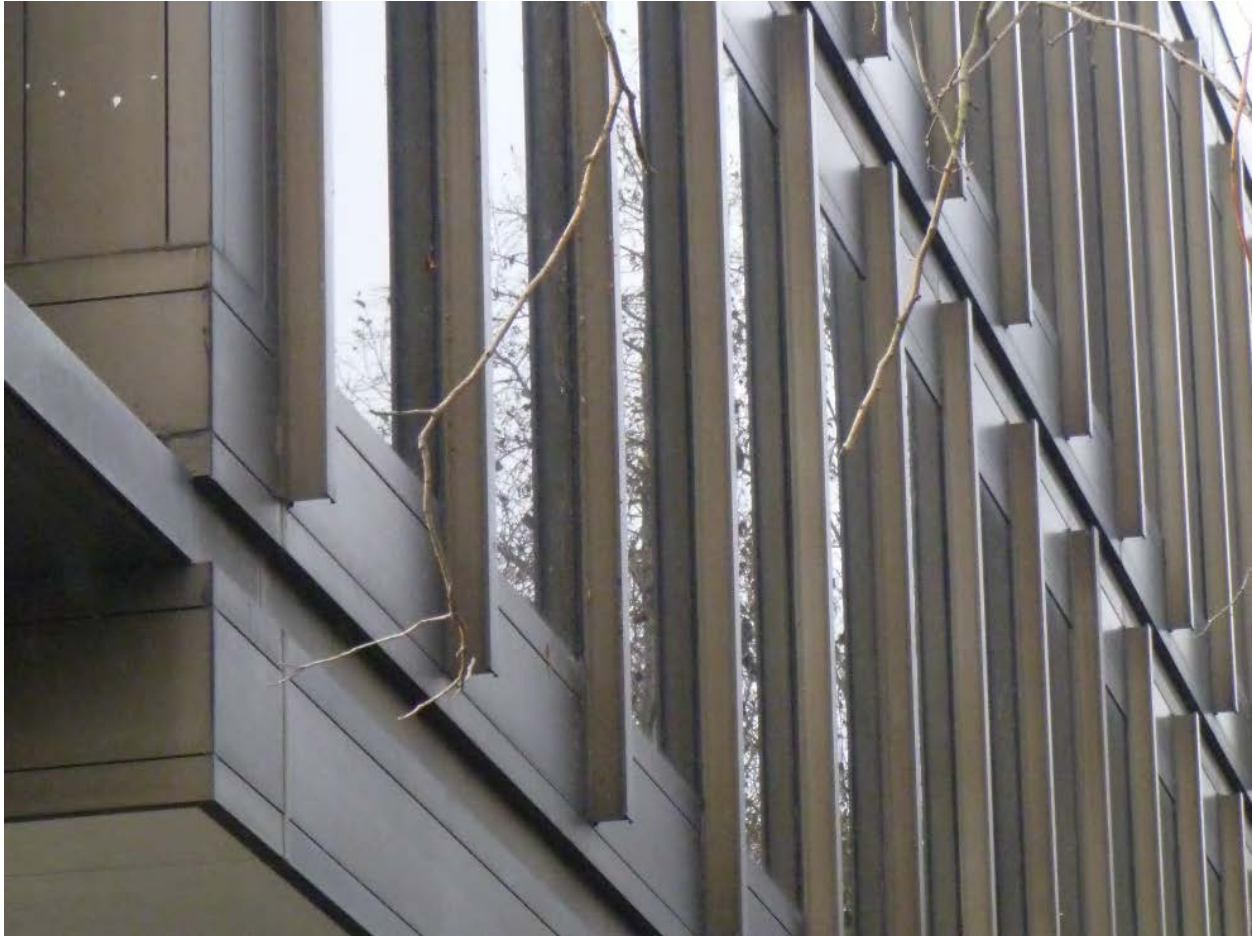
Figure 5. Curtain wall mullions.
