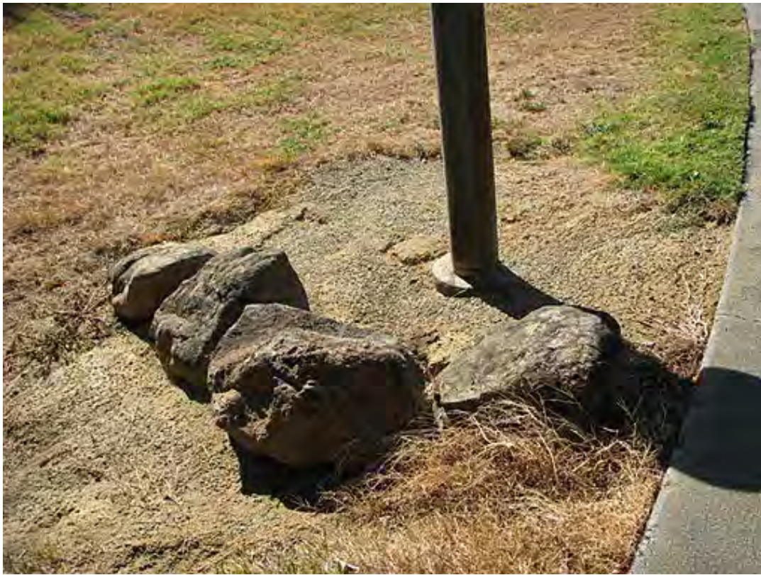
PHOTOGRAPH 21: Stones placed on slope for erosion control.
