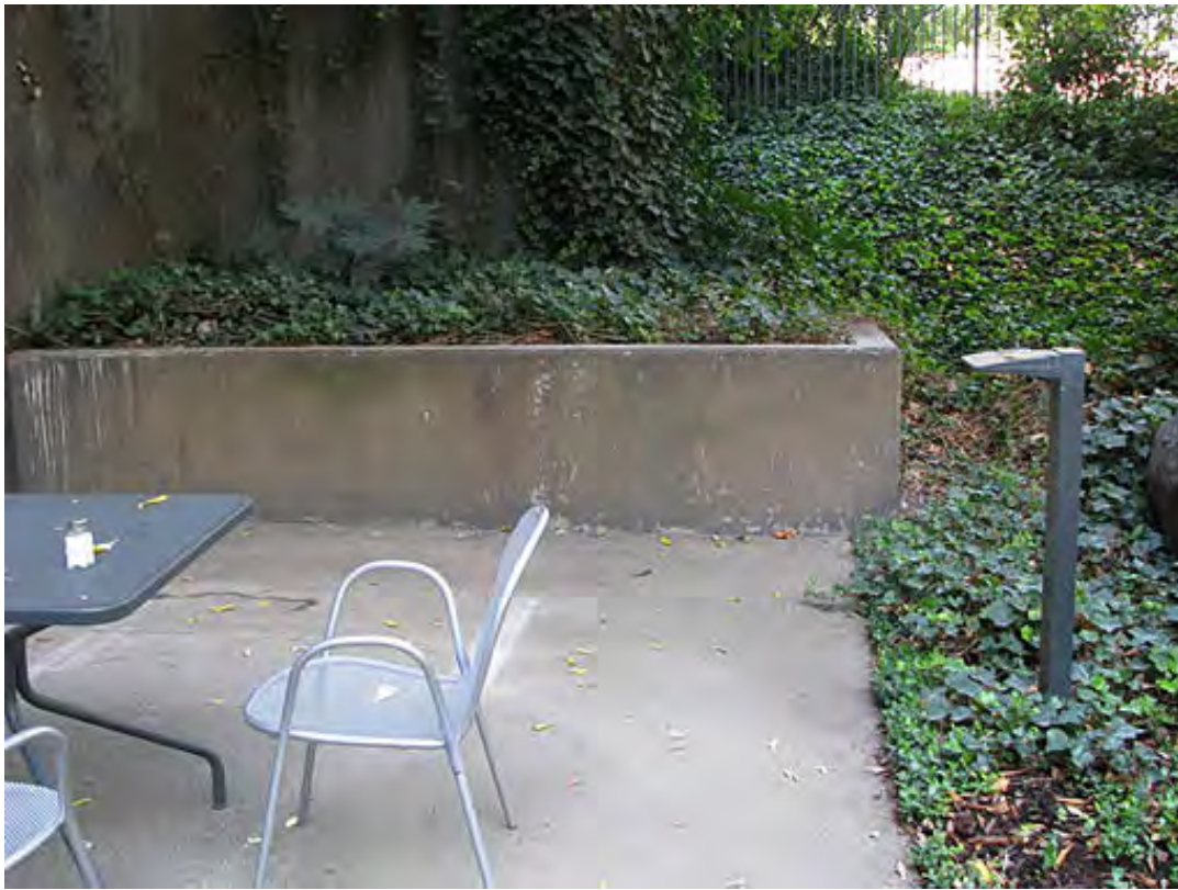
PHOTOGRAPH 67: Concrete retaining wall and slopes at cafeteria terrace.
