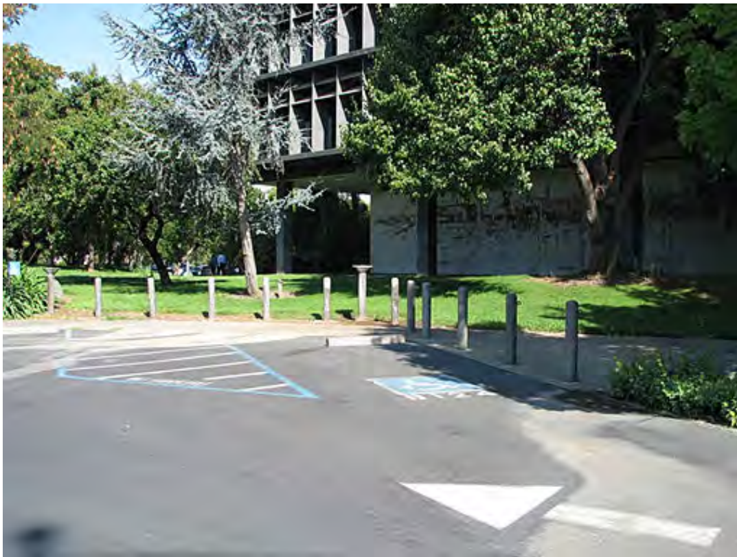
PHOTOGRAPH 8: Parking with new bollards at the south façade of the building.
