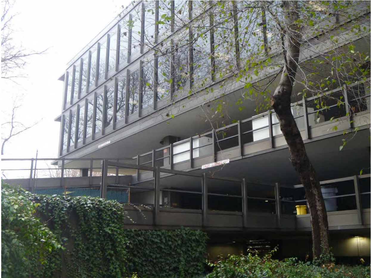
Figure 4. North elevation, office wing over parking garage.
