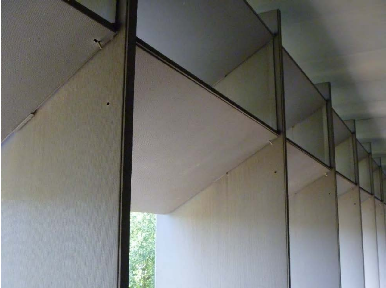
Figure 7. Vertical aluminum fins and horizontal louvers mounted between the brise soleil.
