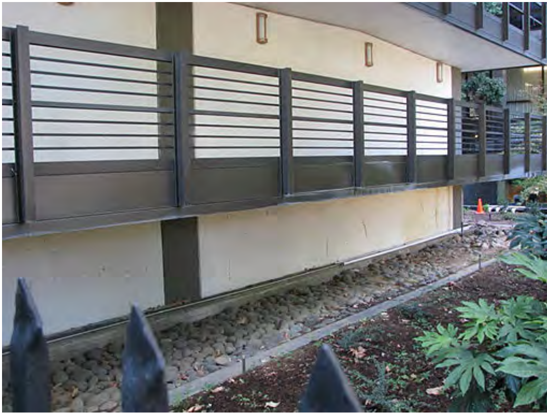
PHOTOGRAPH 45: Elevated outdoor walkway near the cafeteria terrace.
