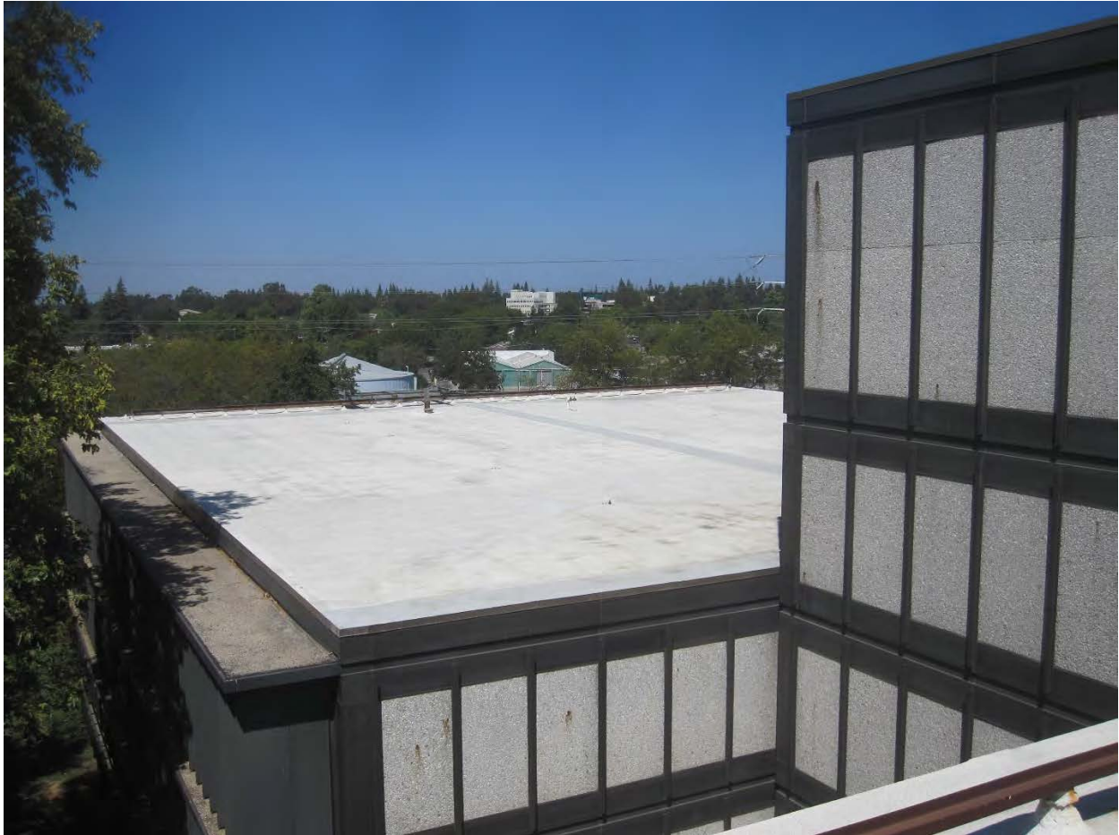
Figure 8. Existing roof at the north wing.
