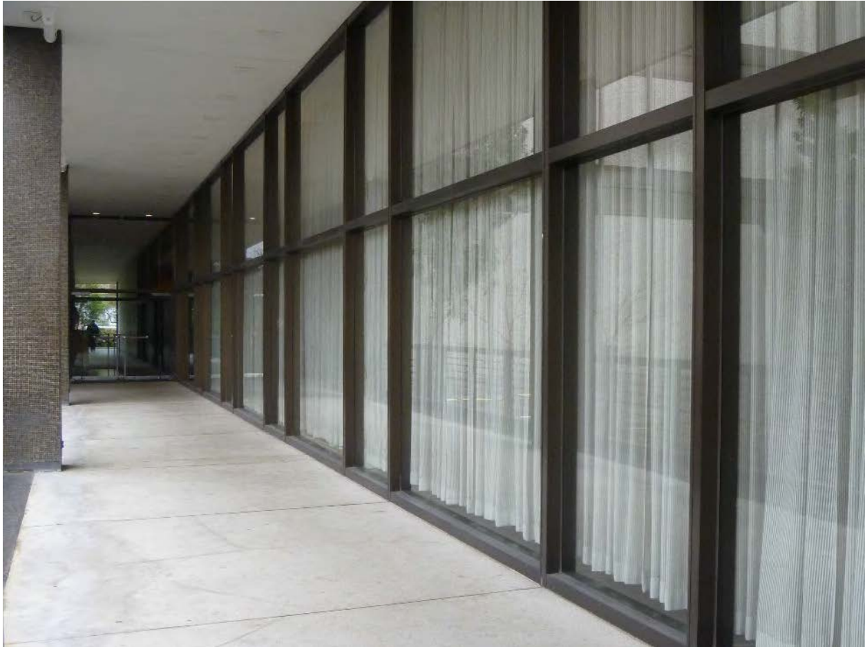
Figure 9. Ground-floor storefront, north elevation of the south wing.
