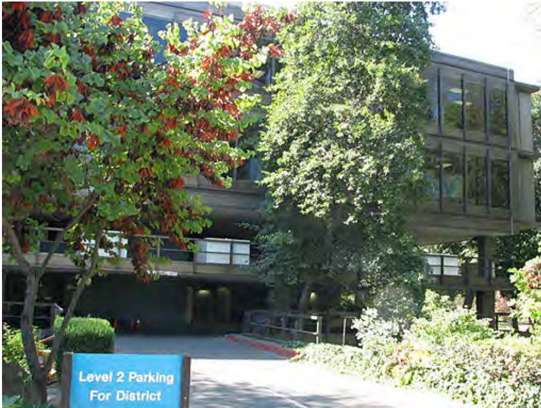
PHOTOGRAPH 52: View of the building's north wing.
