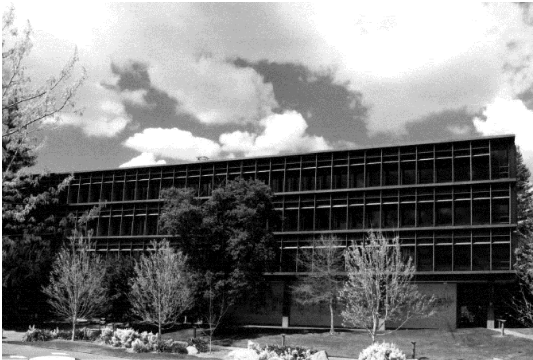
PHOTOGRAPH 13: 2009 Conditions, south façade.
