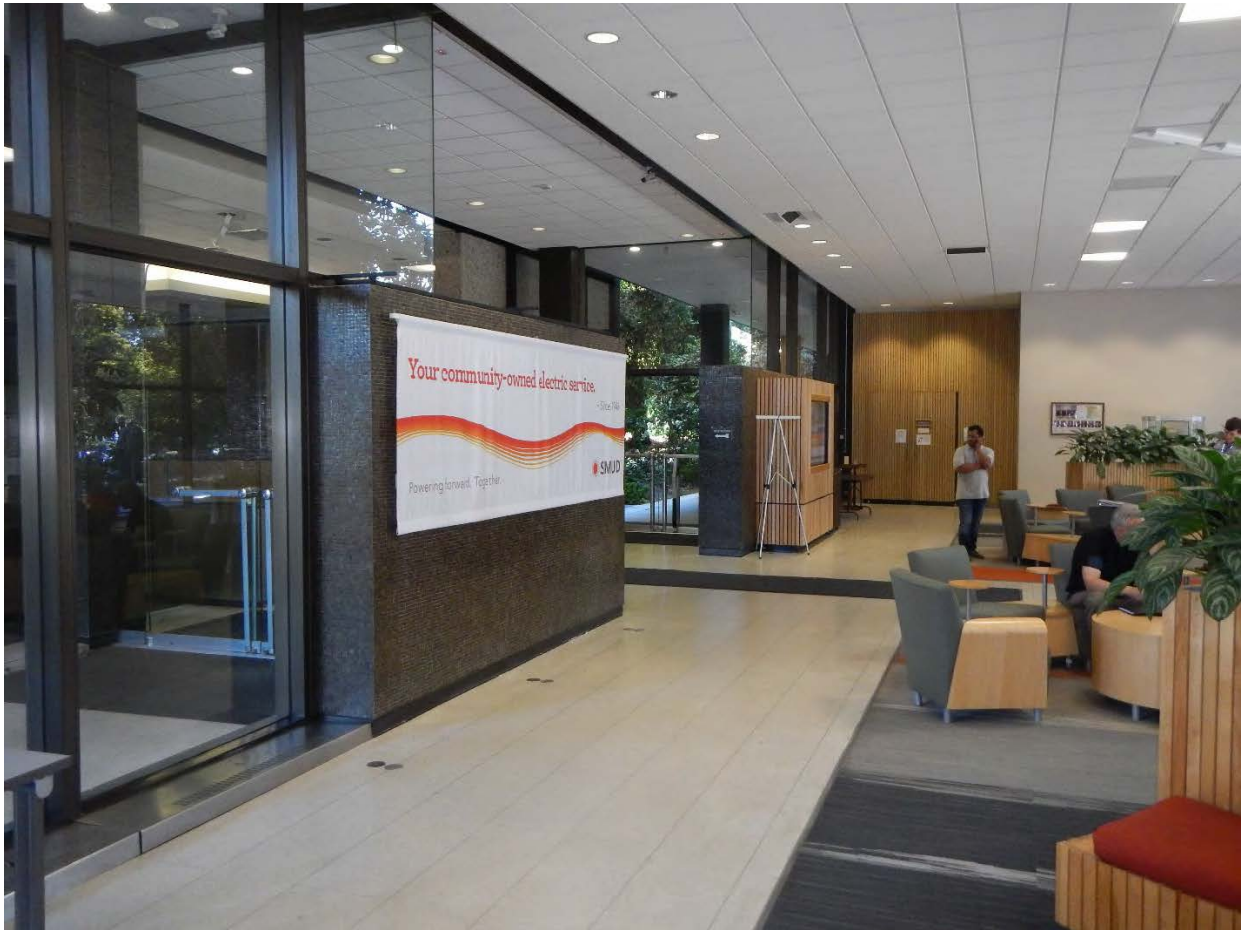
Figure 19. Opening to elevator lobby and curtain walls at the north wall of the lobby. Note the vented steel cap at the base of the curtain wall, and nonoriginal furniture, carpet, and ceiling tiles.
