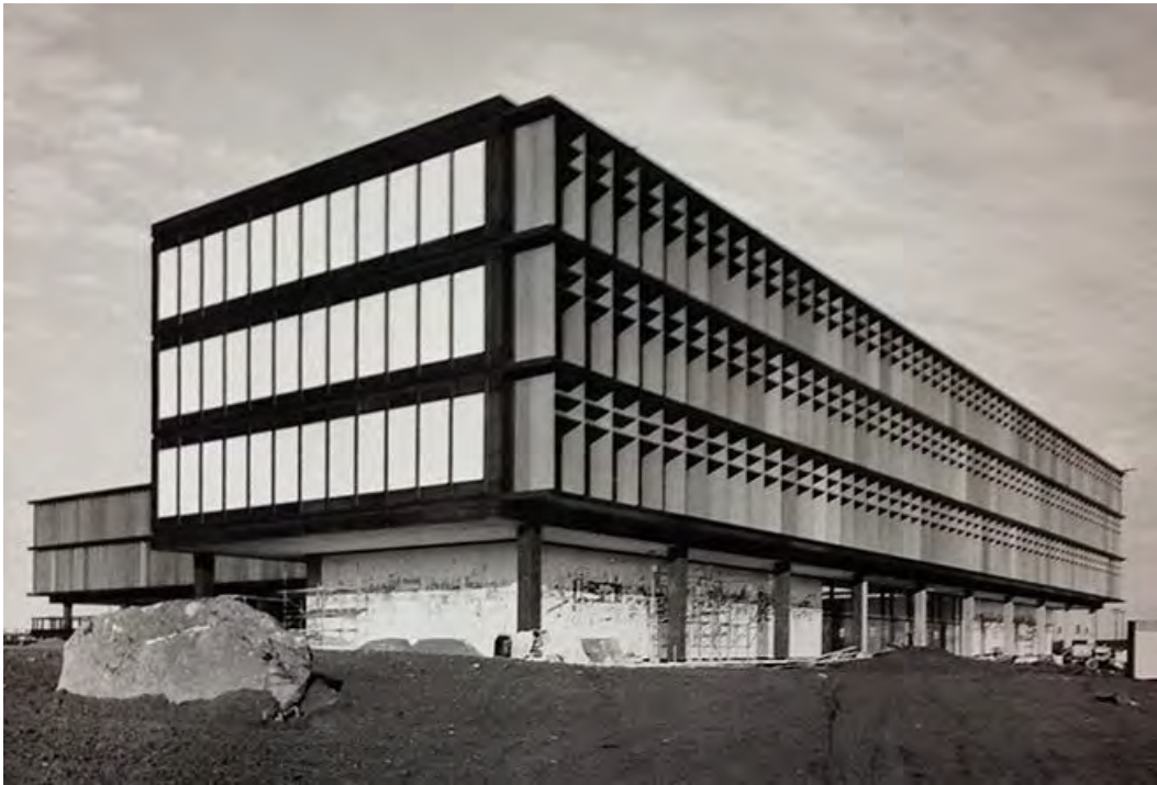
PHOTOGRAPH 3: May 4, 1960 construction showing the south façade of the building, the boulders, and graded site.
