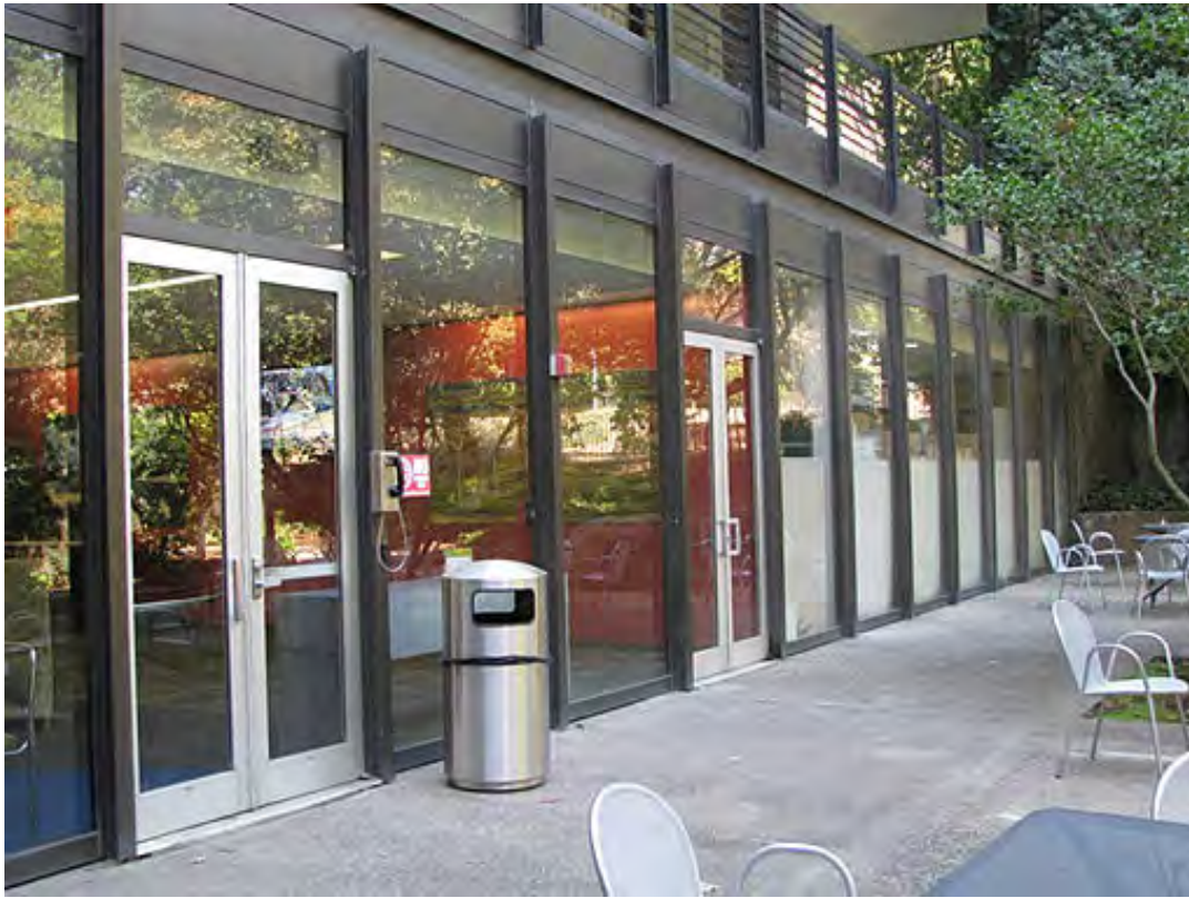
PHOTOGRAPH 72: Glazed walls at cafeteria terrace.
