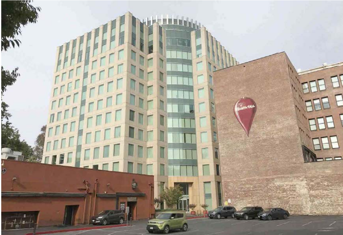
Photo No. 9 View to the southwest of high-rise commercial office building beyond Kayak Alley
