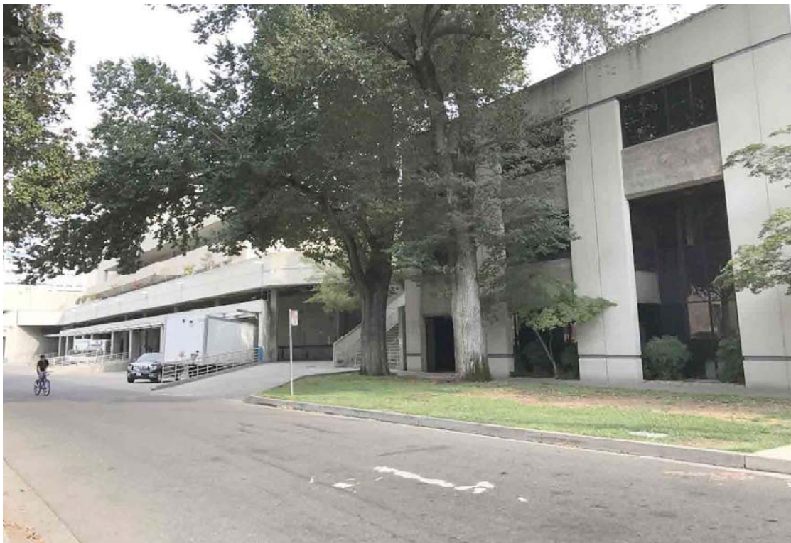
Photo No. 4 View to the northwest of the Sacramento Convention Center beyond K Street
