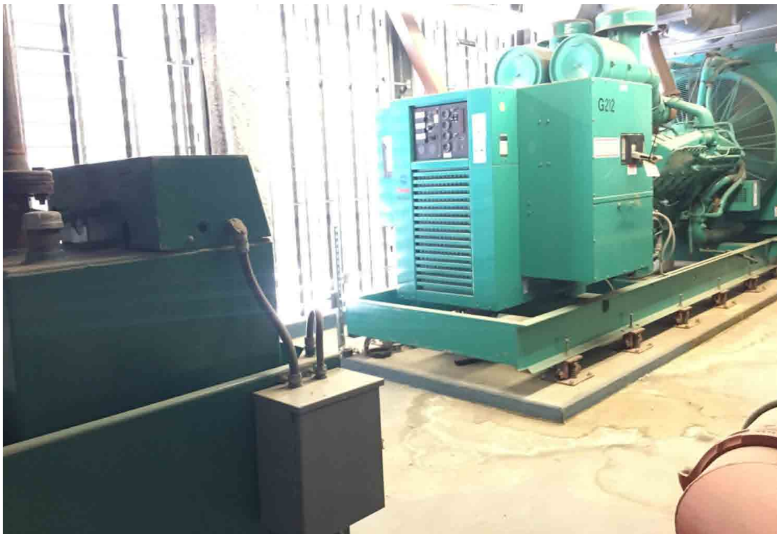
Photo No. 14 Unused/disconnected generator and empty/disconnected diesel holding tank
