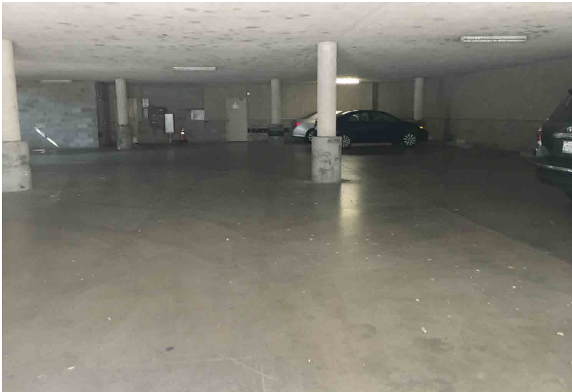
Photo No. 16 Parking garage at 1030 15th Street
