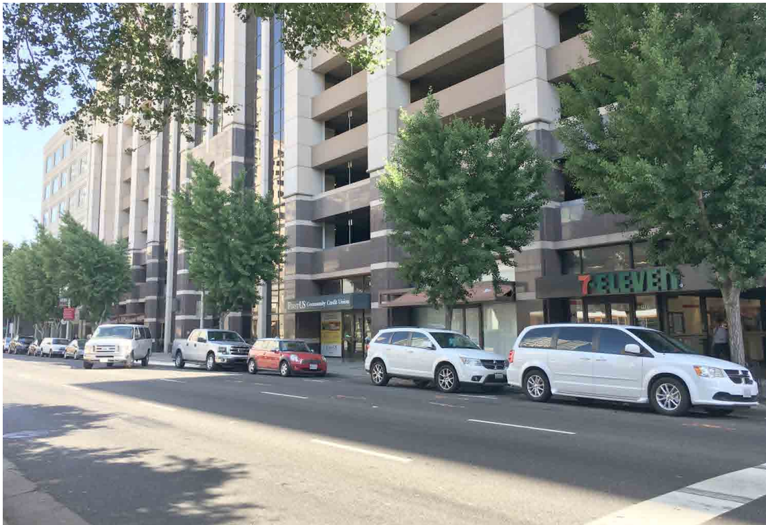
Photo No. 24 View to the north of J Street beyond which are office buildings with commercial/retail storefronts on first floor
