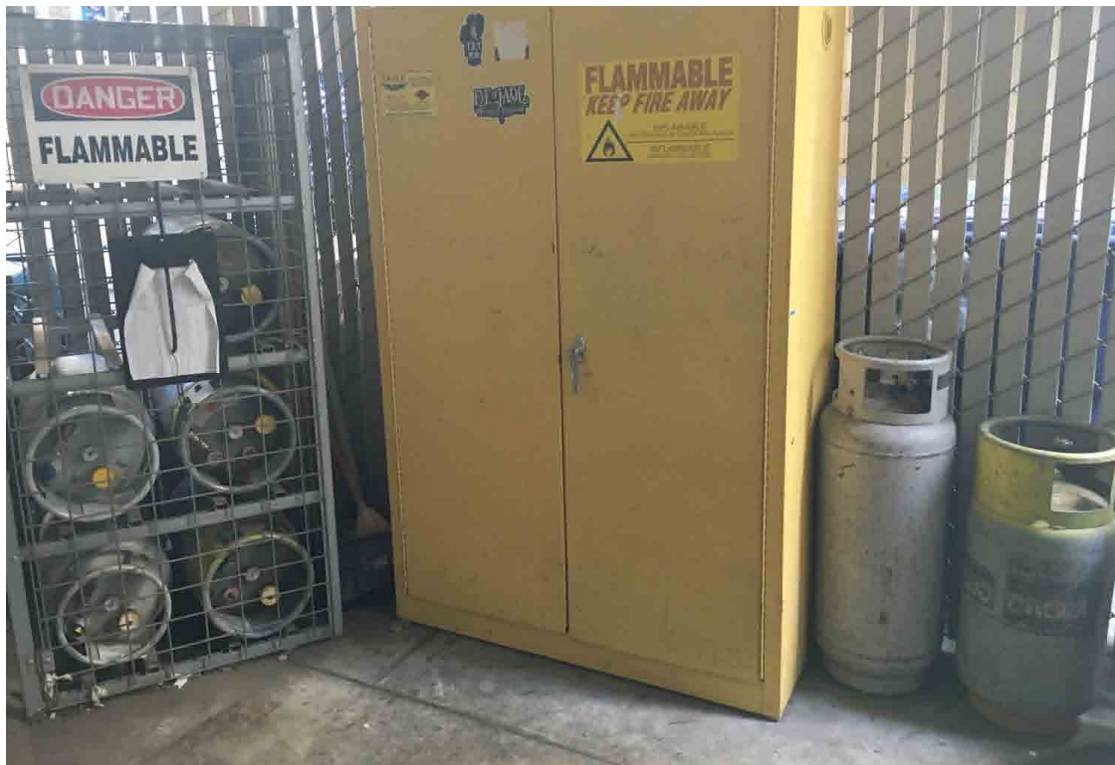
Photo No. 22 Propane and gasoline storage (in steel cabinet < 20 gallons)
