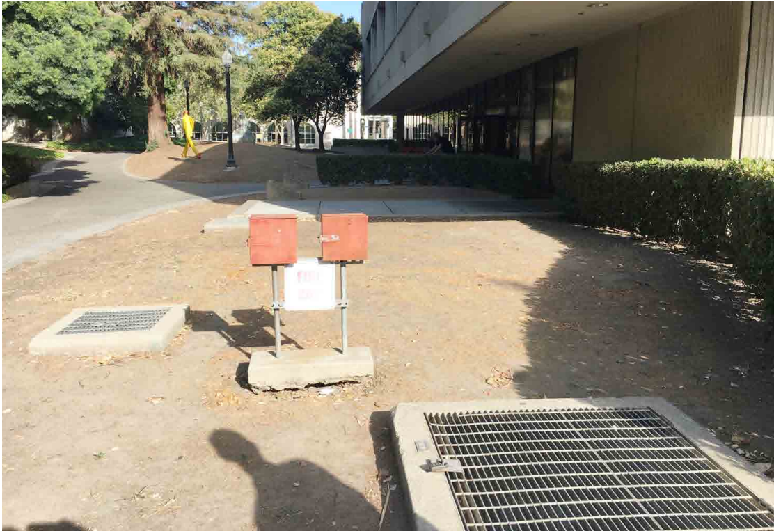
Photo No. 9 Utility vents to basement
