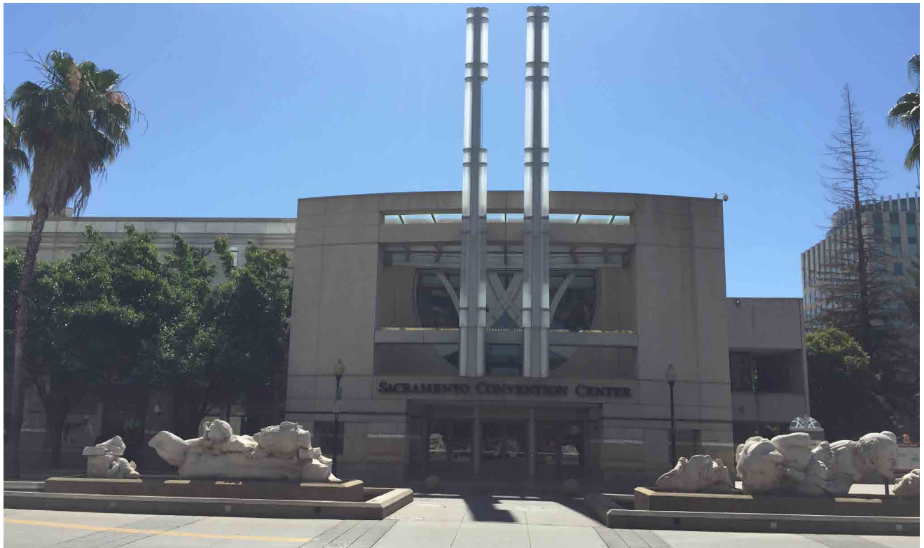
Viewpoint 1: Sacramento Convention Center (SCC) 13th Street entrance. View facing east.
