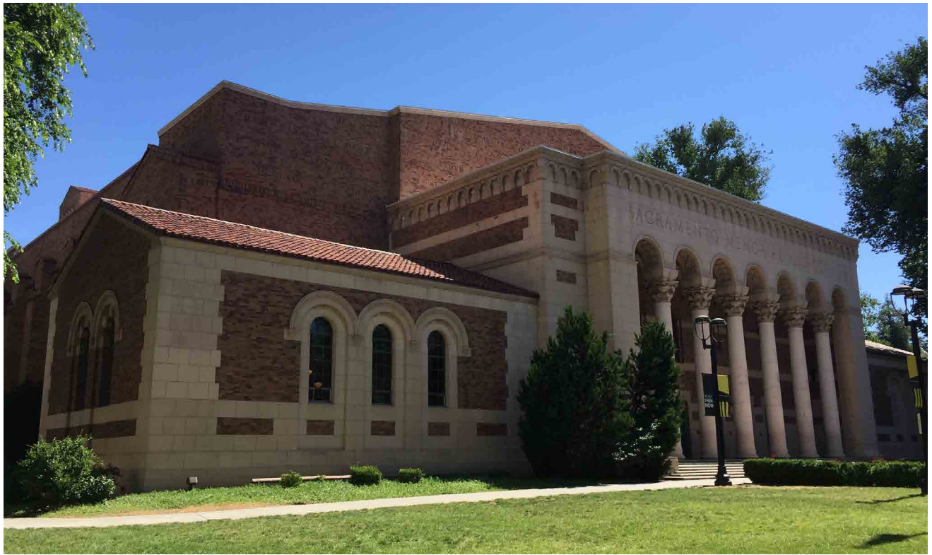
Viewpoint 13: Sacramento Memorial Auditorium. View facing northeast
