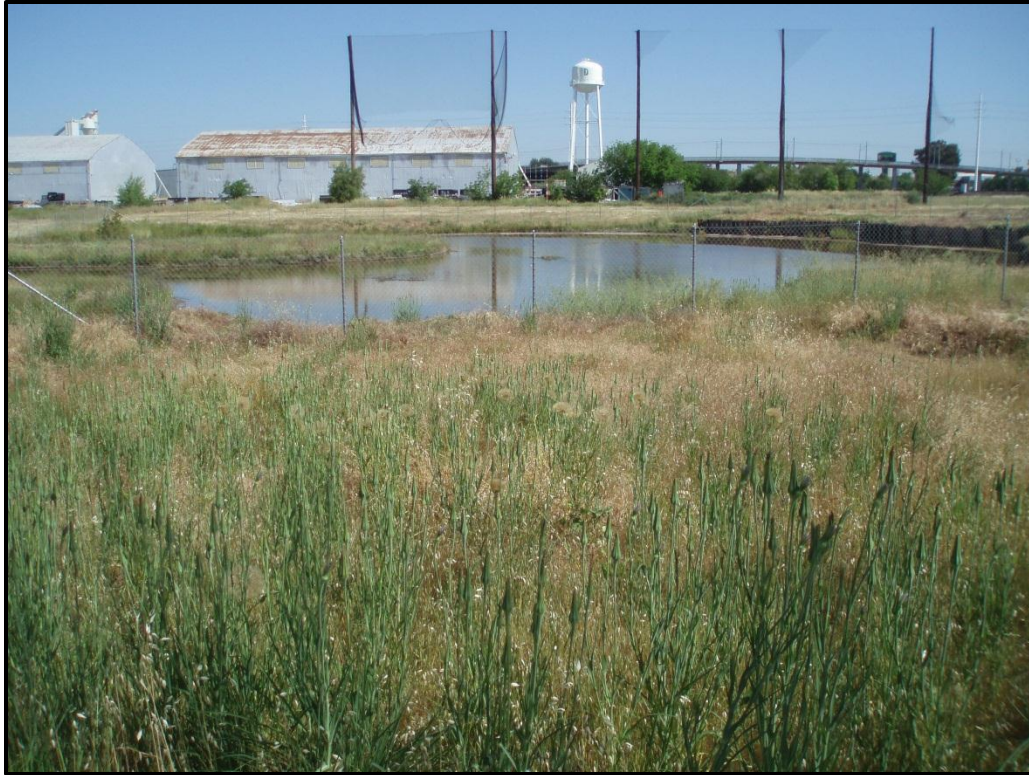
Photo 3 – Concrete Lined Pond Looking North
