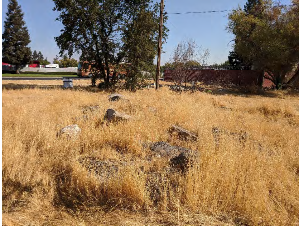
Photo 3: View of piles of concrete and fill located in the northwestern corner of the Study Area. Photo taken September 22, 2021.
